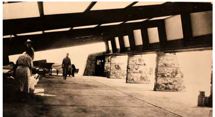
Figure 8-2 - Interior of the Drafting Studio ca. 1939 (The Frank Lloyd Wright Foundation Archives, The Museum of Modern Art | Avery Architectural & Fine Arts Library, Columbia University, New York).
