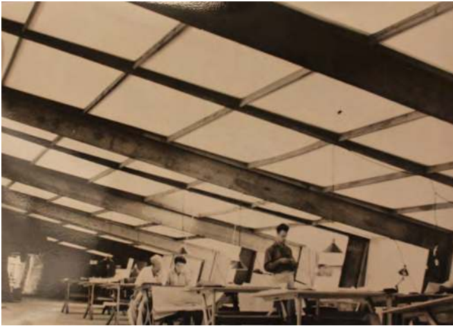
Figure 6-7 - Canvas roof overhead in Drafting Studio, ca. 1939 (The Frank Lloyd Wright Foundation Archives, The Museum of Modern Art | Avery Architectural & Fine Arts Library, Columbia University, New York).
