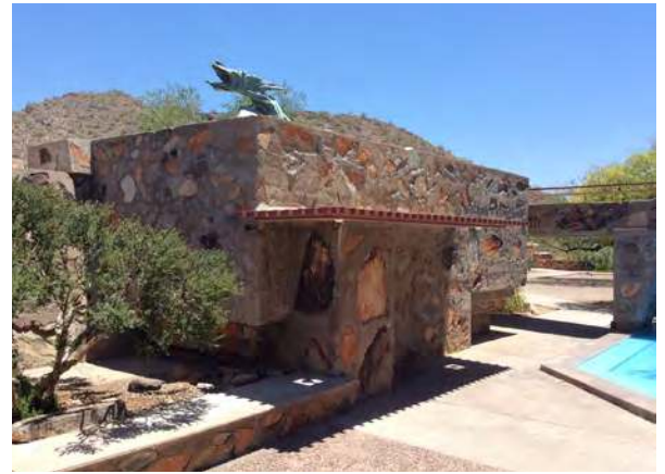
Figure 8-12 - Kiva - Zone 1 (Harboe Architects)
