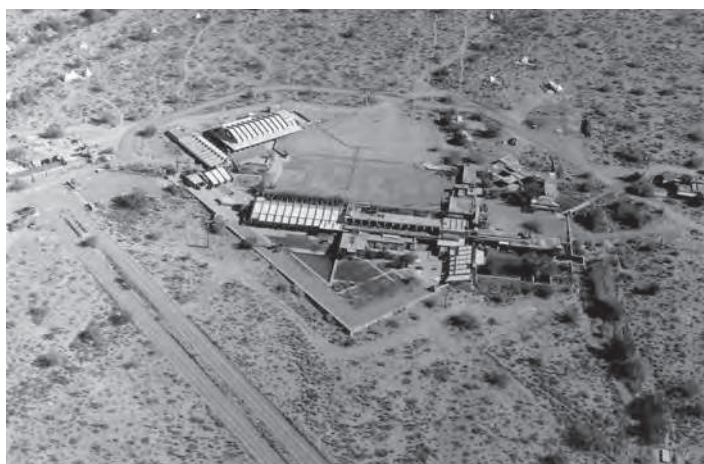
Figure 6-16 - Aerial view of Taliesin West showing new entry drive and area cleared for orchard, 1959 (Pedro Guerrero)
