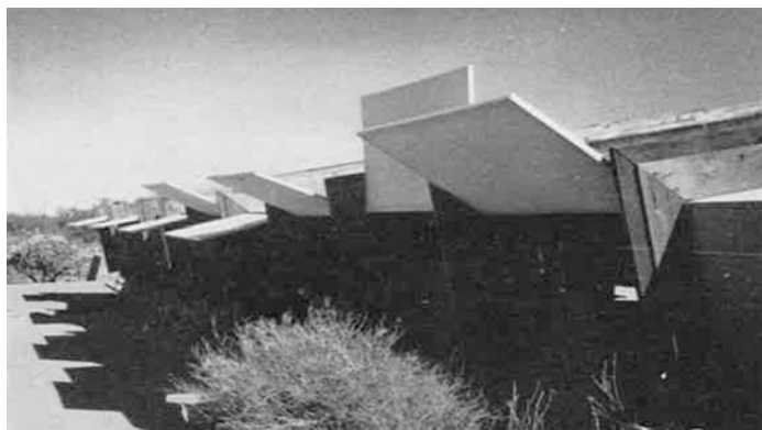
Figure 8-3 - Operable canvas panels on the Drafting Studio, ca. 1939 (The Frank Lloyd Wright Foundation Archives, The Museum of Modern Art | Avery Architectural & Fine Arts Library, Columbia University, New York).
