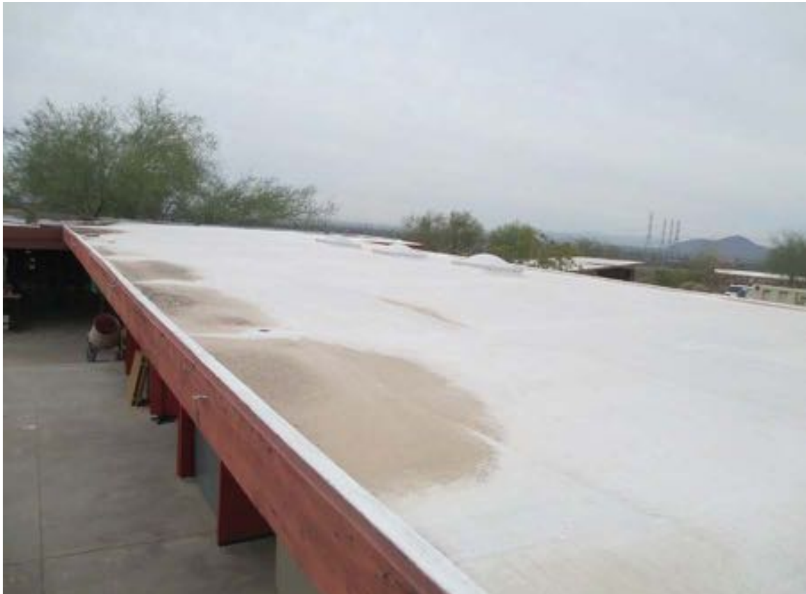
Figure 11-134 - View of Shops roof, 2014 (Harboe Architects).
