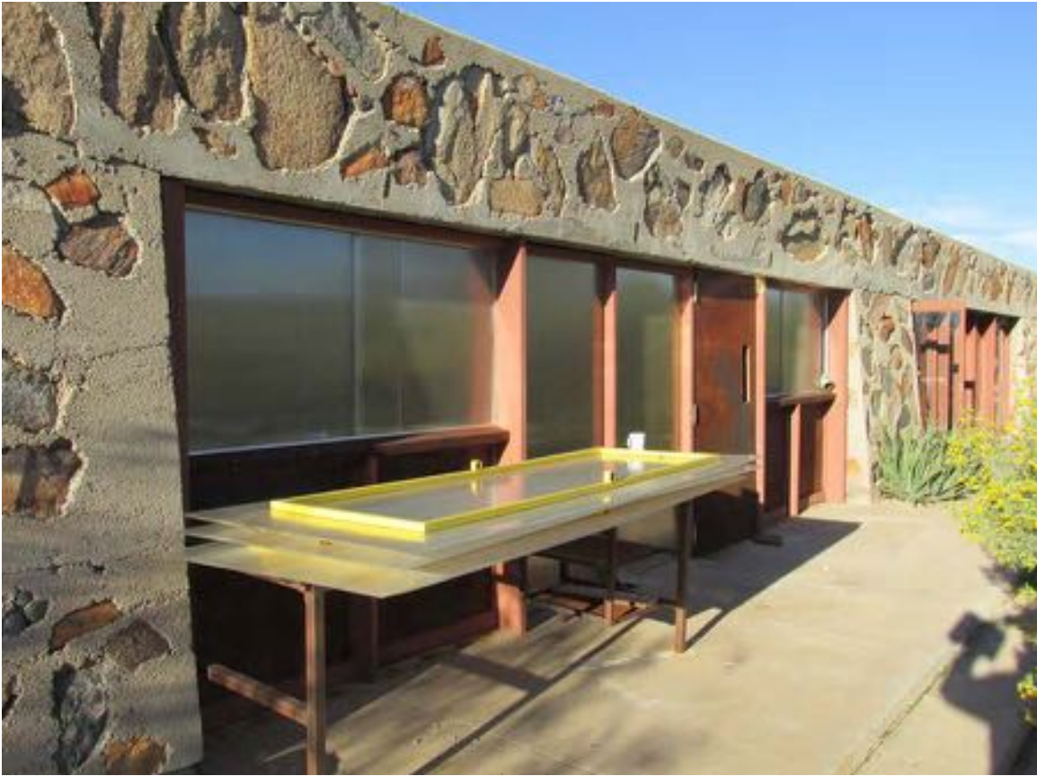
Figure 10-227 - North side of East Wing, 2015 (Harboe Architects).
