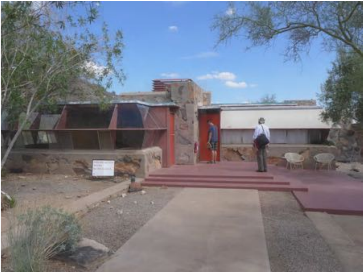
Figure 11-151 - Looking northeast at Sun Cottage, 2014 (Harboe Architects).
