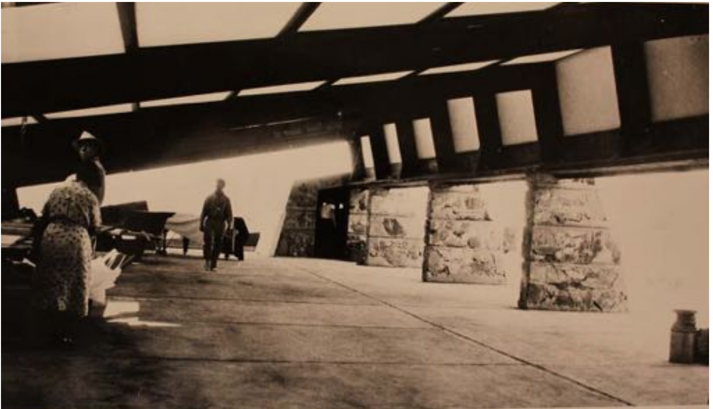
Figure 7-8 - Inside Drafting Studio looking northwest, ca. 1939 (The Frank Lloyd Wright Foundation Archives, The Museum of Modern Art | Avery Architectural & Fine Arts Library, Columbia University, New York).
