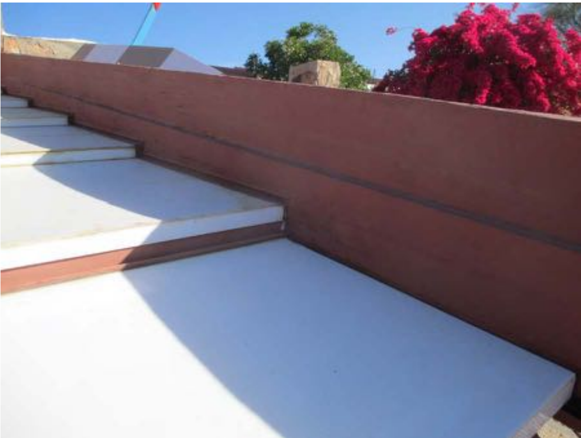
Figure 10-8 - Roof on the office in 2014 (Harboe Architects).
