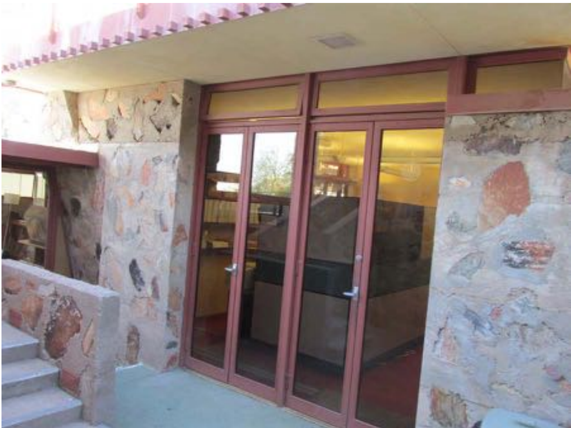
Figure 11-191 - Exterior of Finance Office (Harboe Architects).
