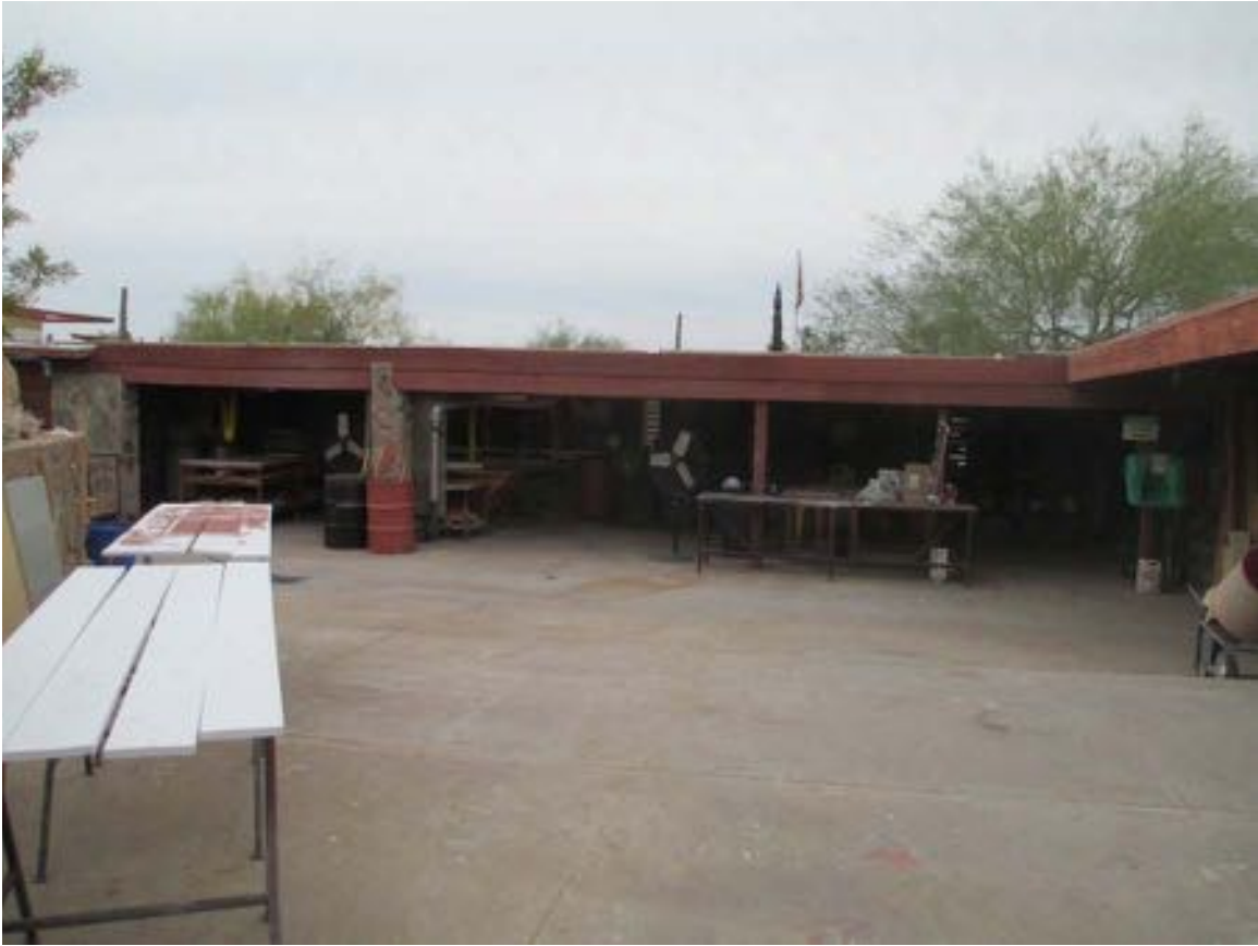
Figure 11-133 - View of Shops looking south, 2014 (Harboe Architects).
