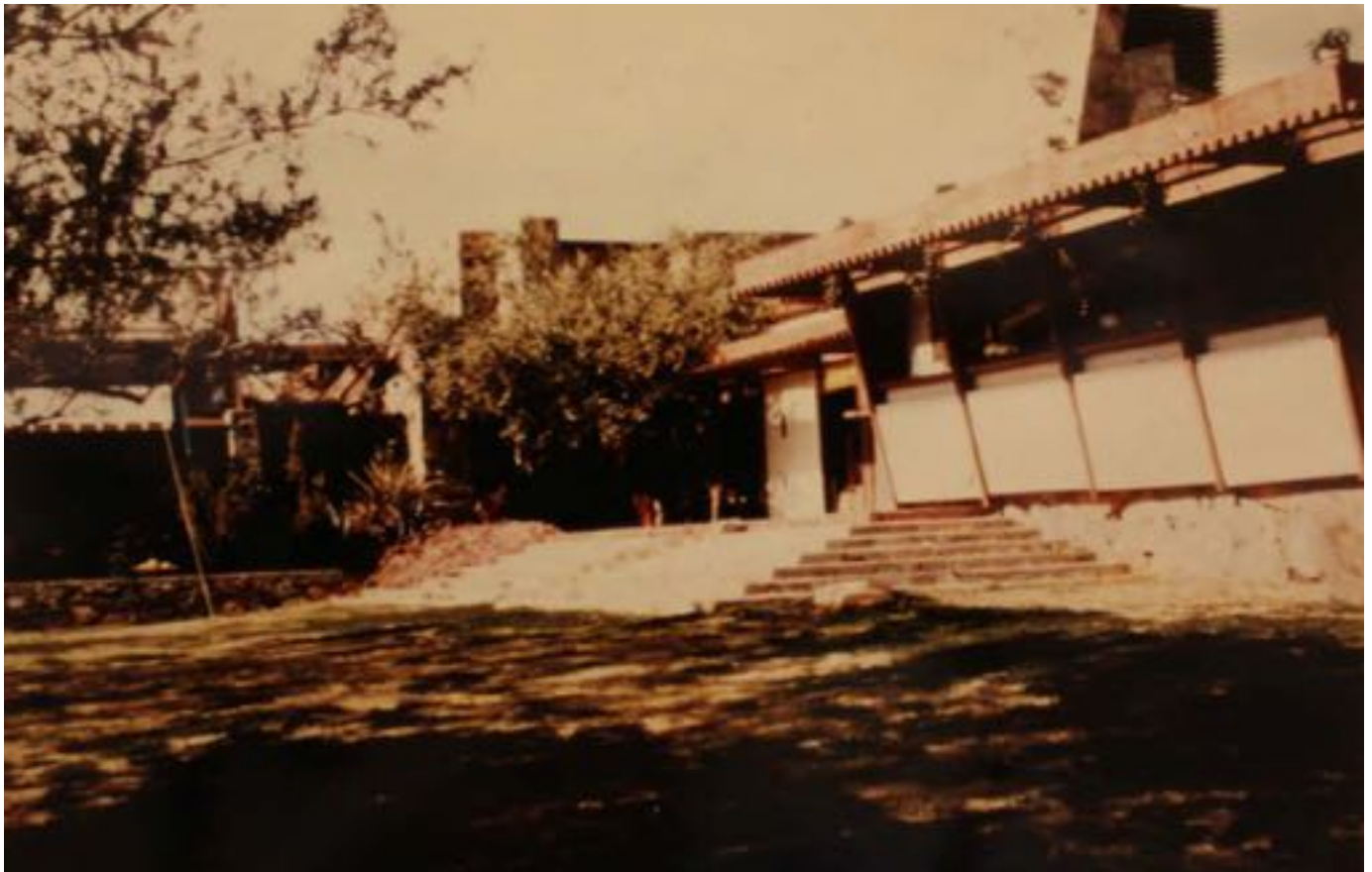
Figure 7-45 - View of Wright's Living Quarters from the garden, ca. 1950 (The Frank Lloyd Wright Foundation Archives, The Museum of Modern Art | Avery Architectural & Fine Arts Library, Columbia University, New York).
