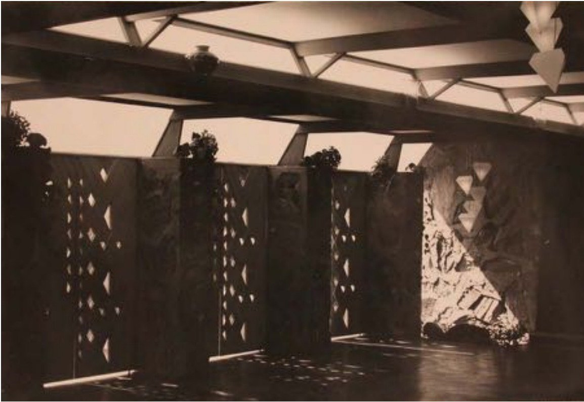
Figure 11-179 - Interior of Atrium looking at decorative concrete and glass panels, ca. 1962 (The Frank Lloyd Wright Foundation Archives, The Museum of Modern Art | Avery Architectural & Fine Arts Library, Columbia University, New York).
