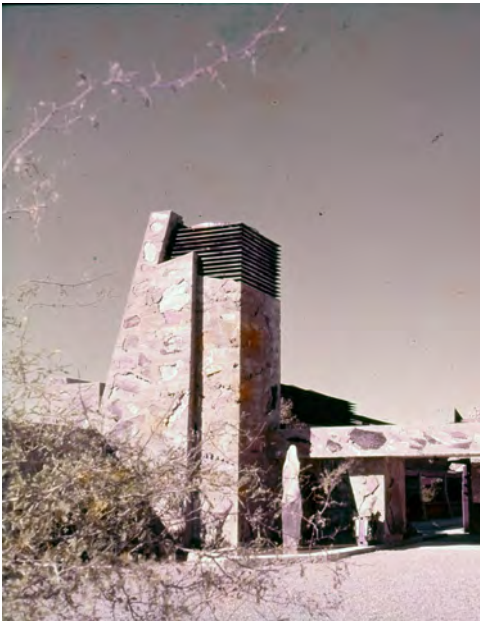
Figure 7-48 - Water Tower ca. 1950 (The Frank Lloyd Wright Foundation Archives, The Museum of Modern Art | Avery Architectural & Fine Arts Library, Columbia University, New York).
