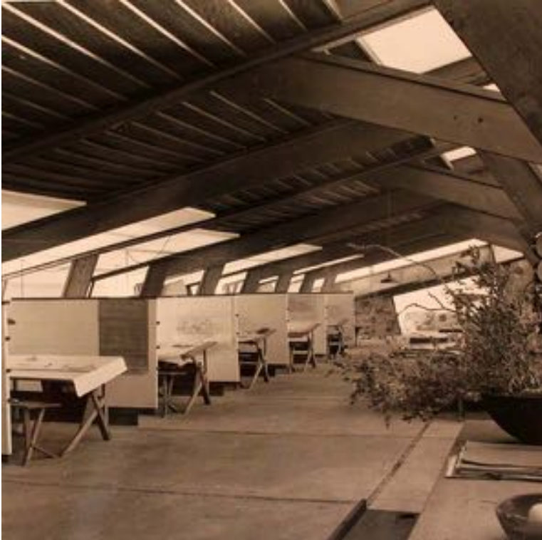
Figure 7-9 - Inside Drafting Studio with wood boards at the center of the ceiling, ca. 1941 (The Frank Lloyd Wright Foundation Archives, The Museum of Modern Art | Avery Architectural & Fine Arts Library, Columbia University, New York).
