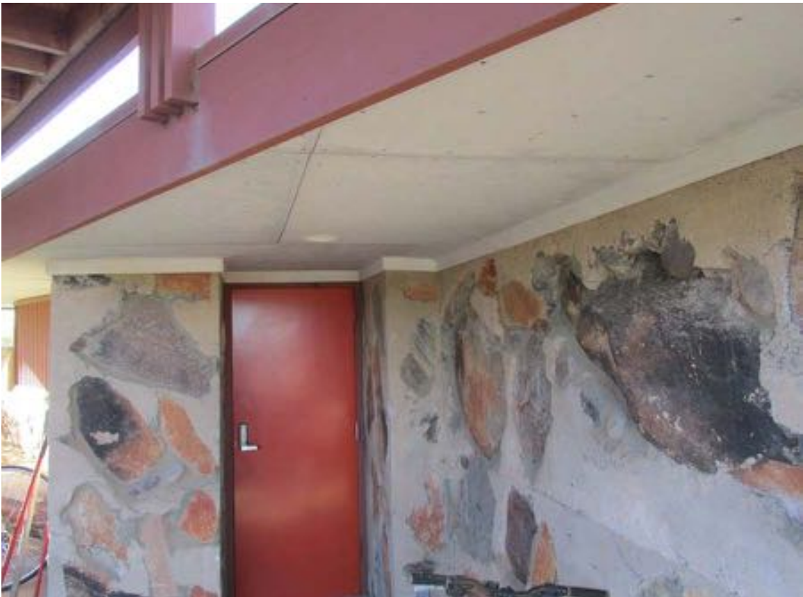
Figure 10-147 - Soffit on northeast side of Men's Locker Room, 2015 (Harboe Architects).
