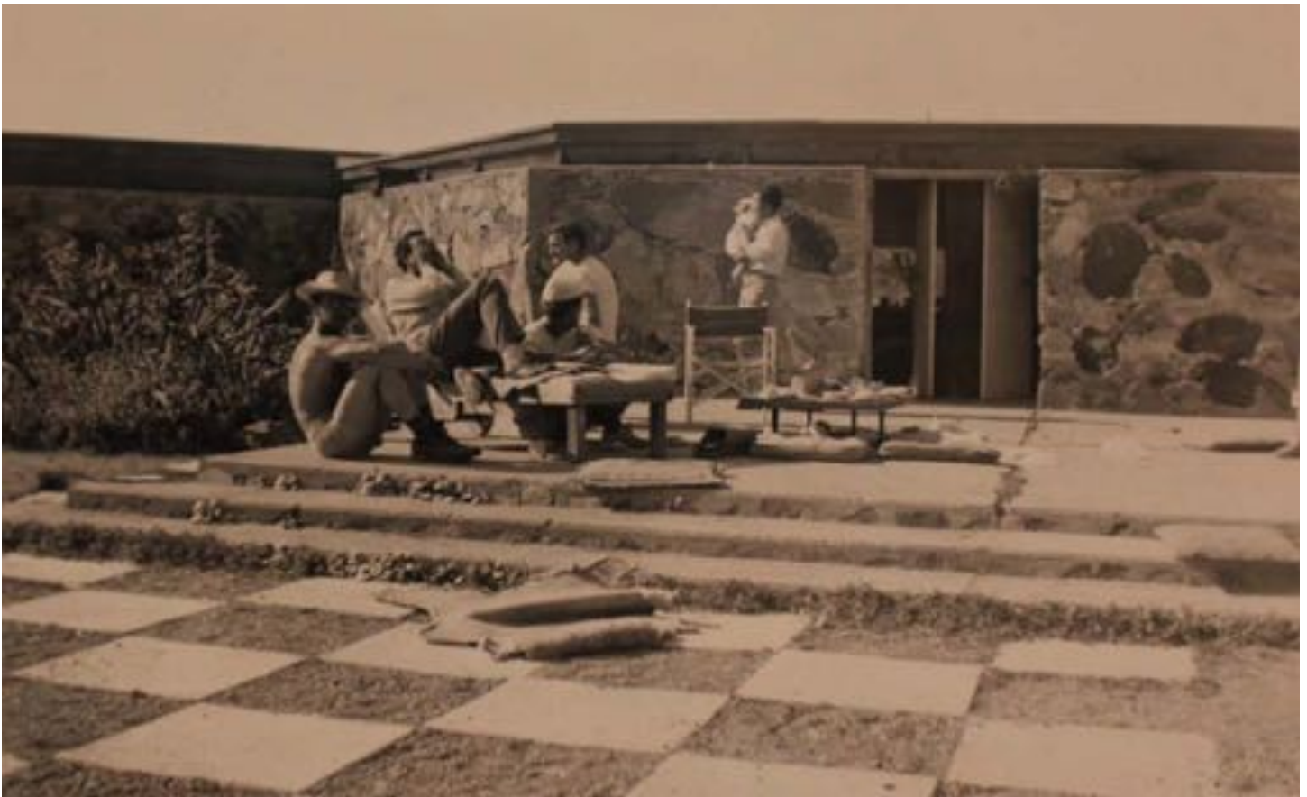
Figure 6-25 - Apprentices Court, ca. 1940 (The Frank Lloyd Wright Foundation Archives, The Museum of Modern Art | Avery Architectural & Fine Arts Library, Columbia University, New York).
