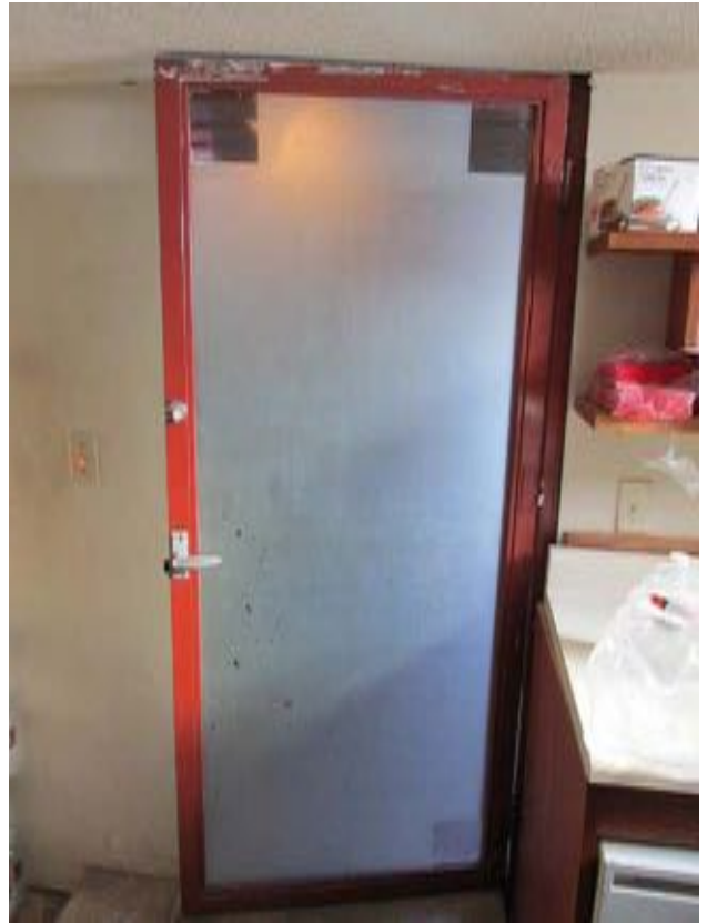
Figure 10-82 - Metal and glass door in the kitchen, 2015 (Harboe Architects).
