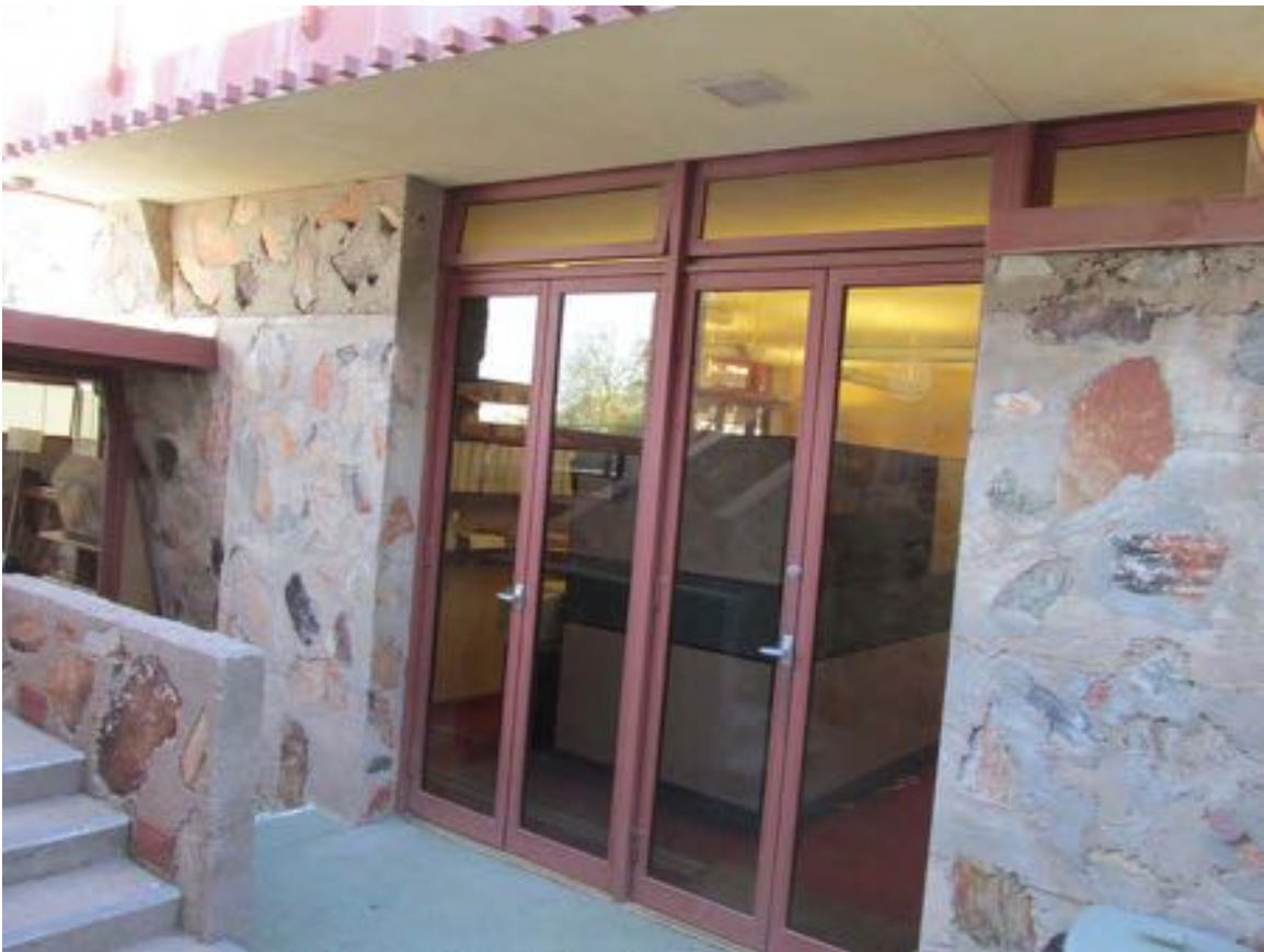
Figure 10-232 - Exterior of Finance Offices, 2015 (Harboe Architects).
