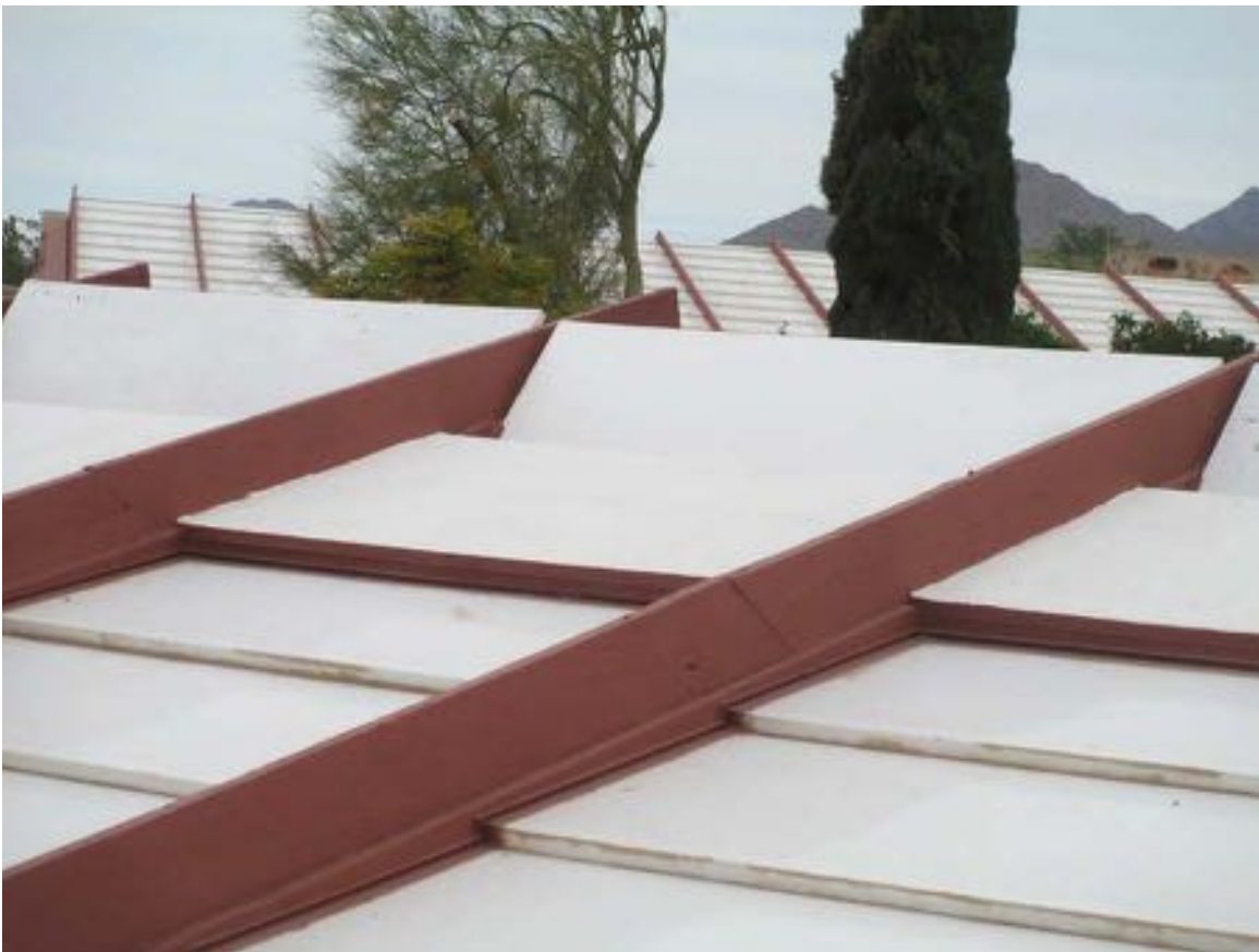
Figure 10-20 - Drafting studio roof, 2014 (Harboe Architects).
