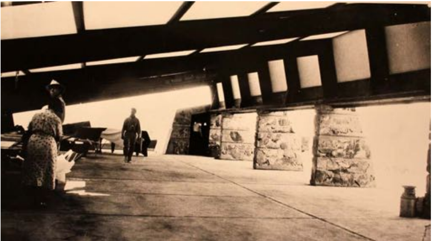
Figure 6-15 - Inside the Drafting Studio looking west with grand piano in background, ca. 1939 (The Frank Lloyd Wright Foundation Archives, The Museum of Modern Art | Avery Architectural & Fine Arts Library, Columbia University, New York).
