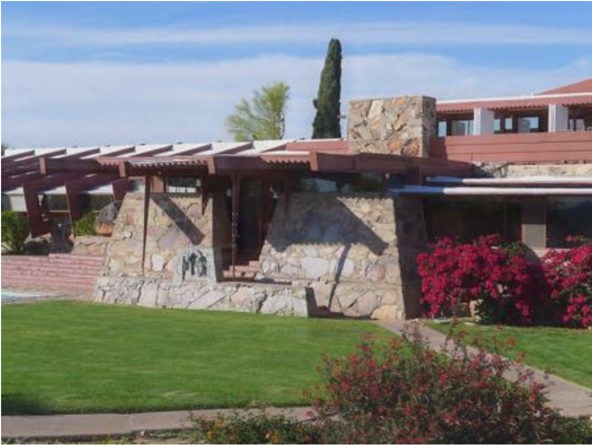
Figure 11-43 - Exterior of Original Dining Room (Board Room) looking north, 2014 (Harboe Architects).
