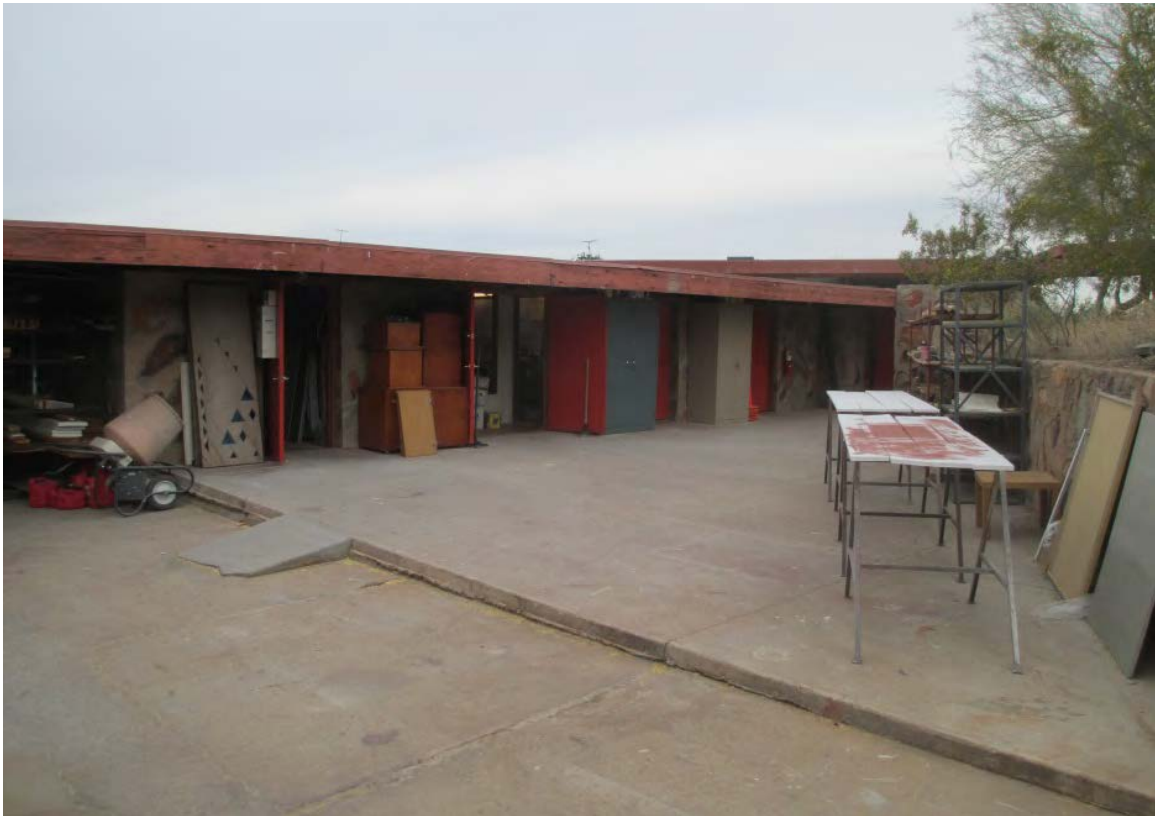
Figure 7-70 - In the courtyard outside the Shops, 2014 (Harboe Architects).
