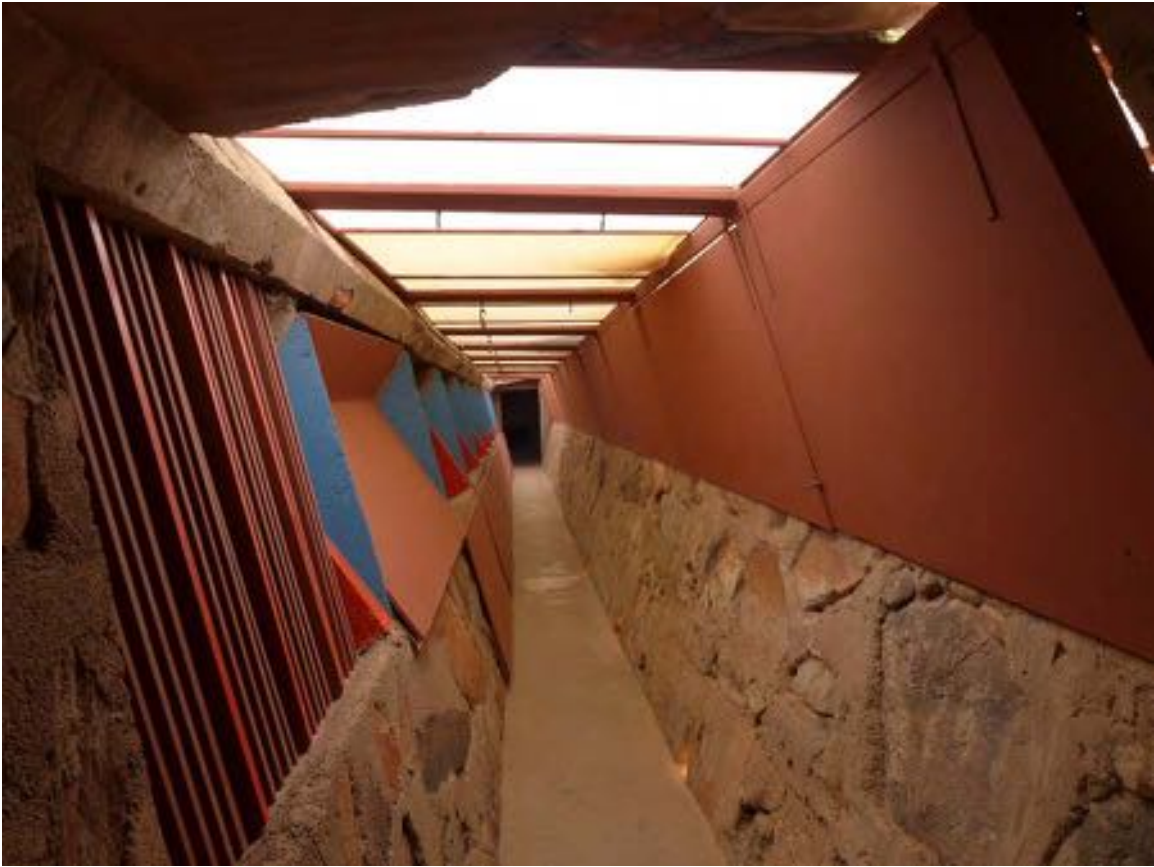
Figure 11-101 - Cabaret corridor looking north, 2014 (Harboe Architects).
