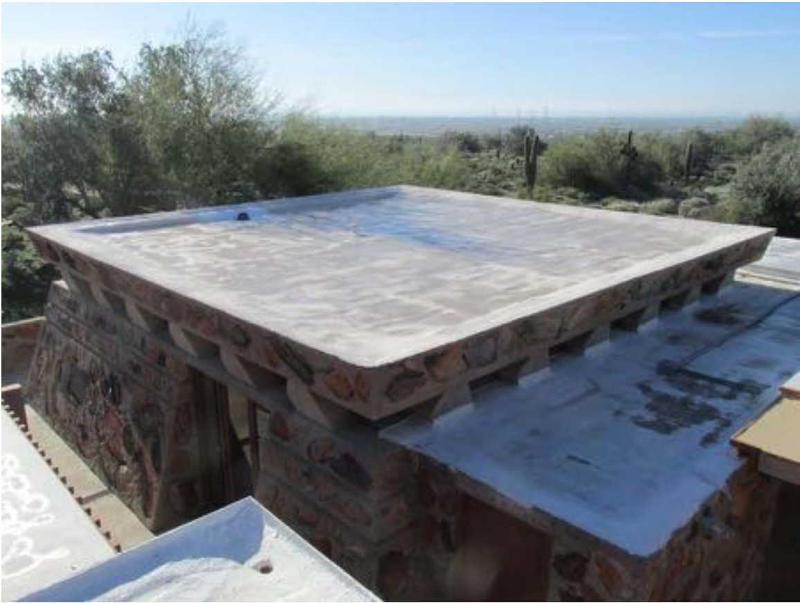
Figure 10-267 - Roof of Clinic Office, 2015 (Harboe Architects).
