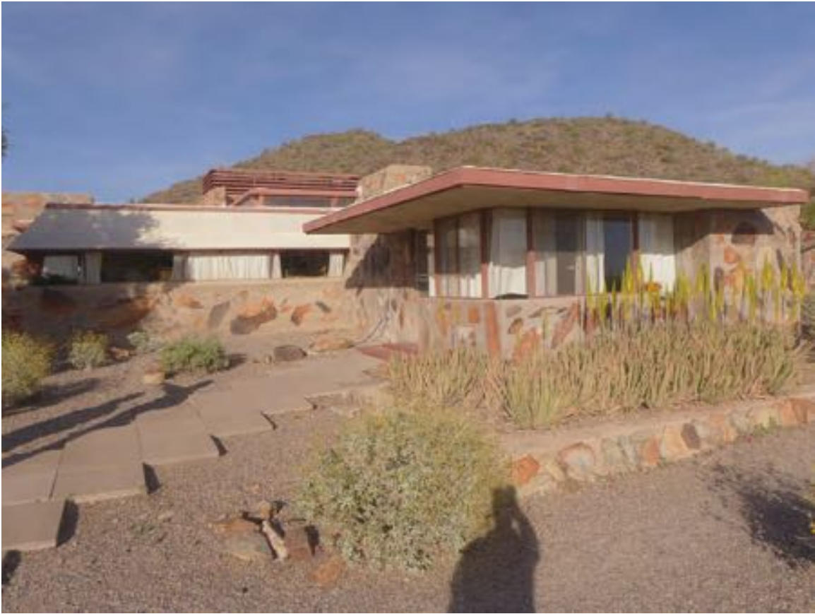
Figure 11-152 - Looking north at Sun Cottage, 2014 (Harboe Architects).
