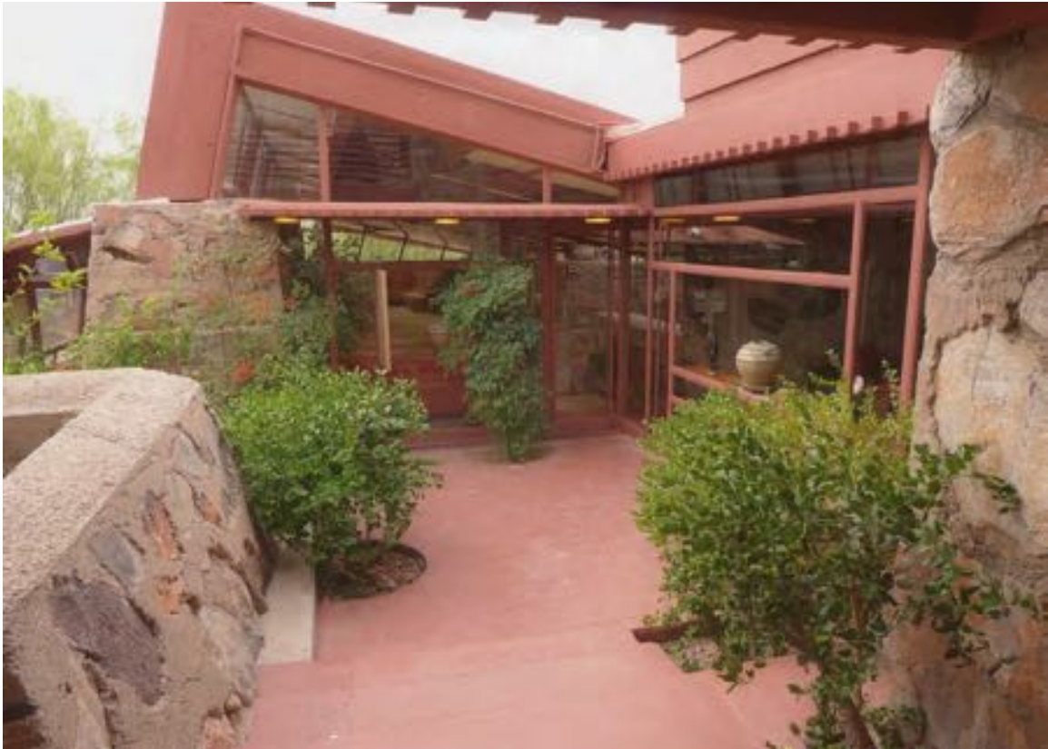
Figure 11-78 - Exterior of Garden Room looking southwest from terrace outside Swan Cove, 2014 (Harboe Architects).
