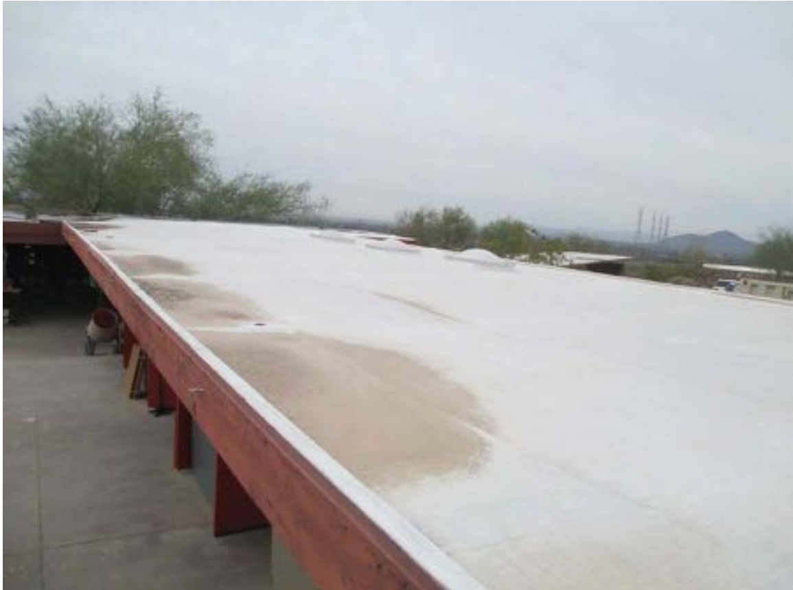
Figure 10-139 - View of Shops roof, 2014 (Harboe Architects).
