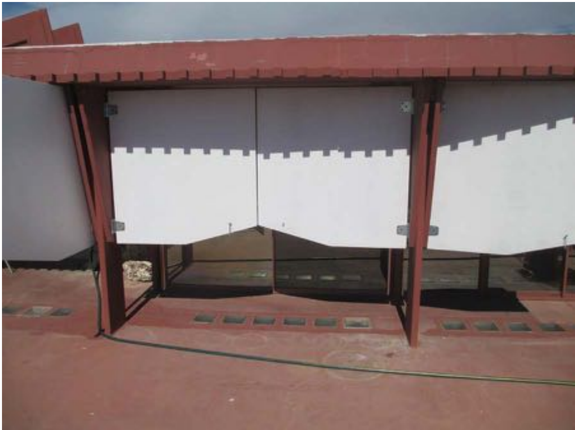
Figure 10-117 - Looking north at guest room with closed wood flaps, 2014 (Harboe Architects).
