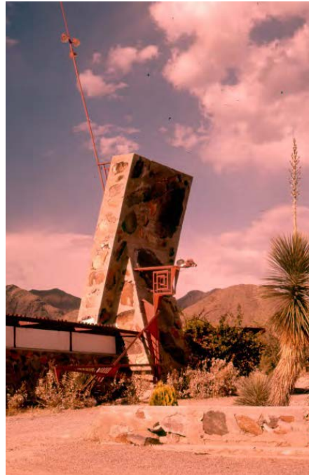
Figure 7-72 - Light Tower, ca. 1955 (The Frank Lloyd Wright Foundation Archives, The Museum of Modern Art | Avery Architectural & Fine Arts Library, Columbia University, New York).
