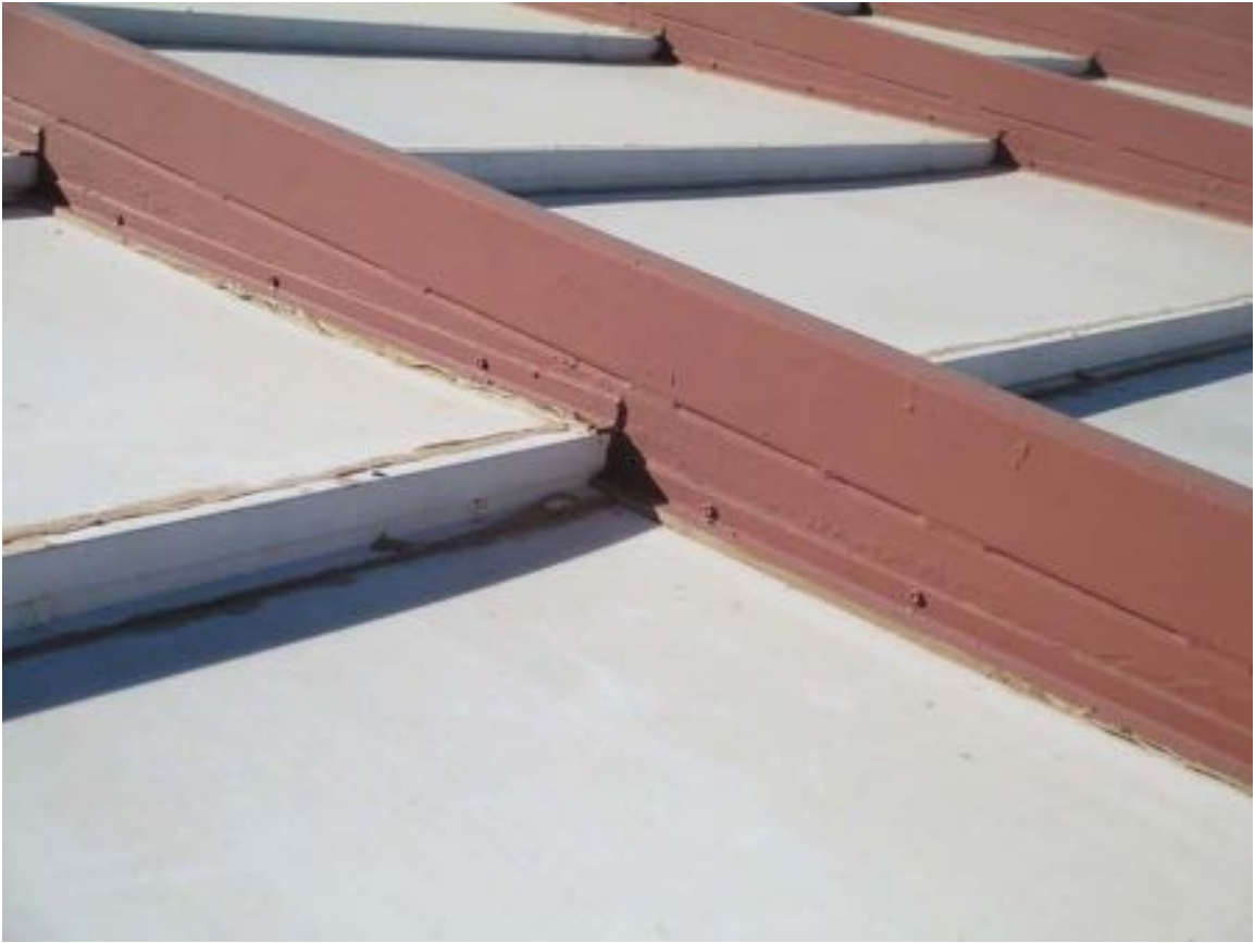
Figure 10-178 - Detail of Pavilion roof, 2014 (Harboe Architects).
