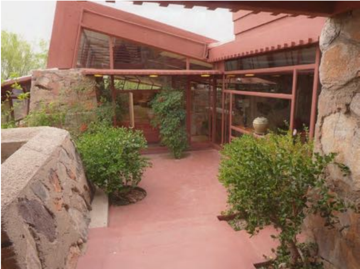
Figure 10-67 - Exterior of Garden Room looking southwest from terrace outside Swan Cove, 2014 (Harboe Architects).
