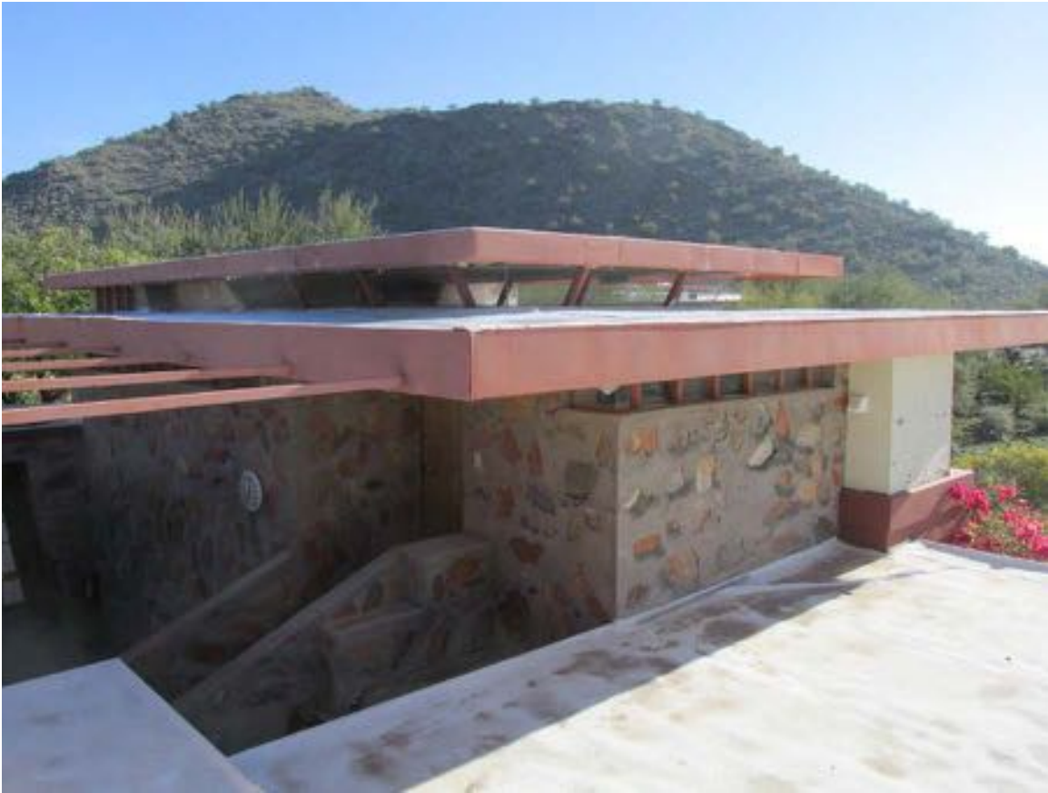
Figure 11-229 - Looking northeast at Tower Office, 2015 (Harboe Architects).
