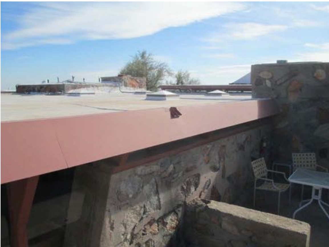
Figure 11-153 - Metal fascia and roof of Sun Cottage, 2014 (Harboe Architects).
