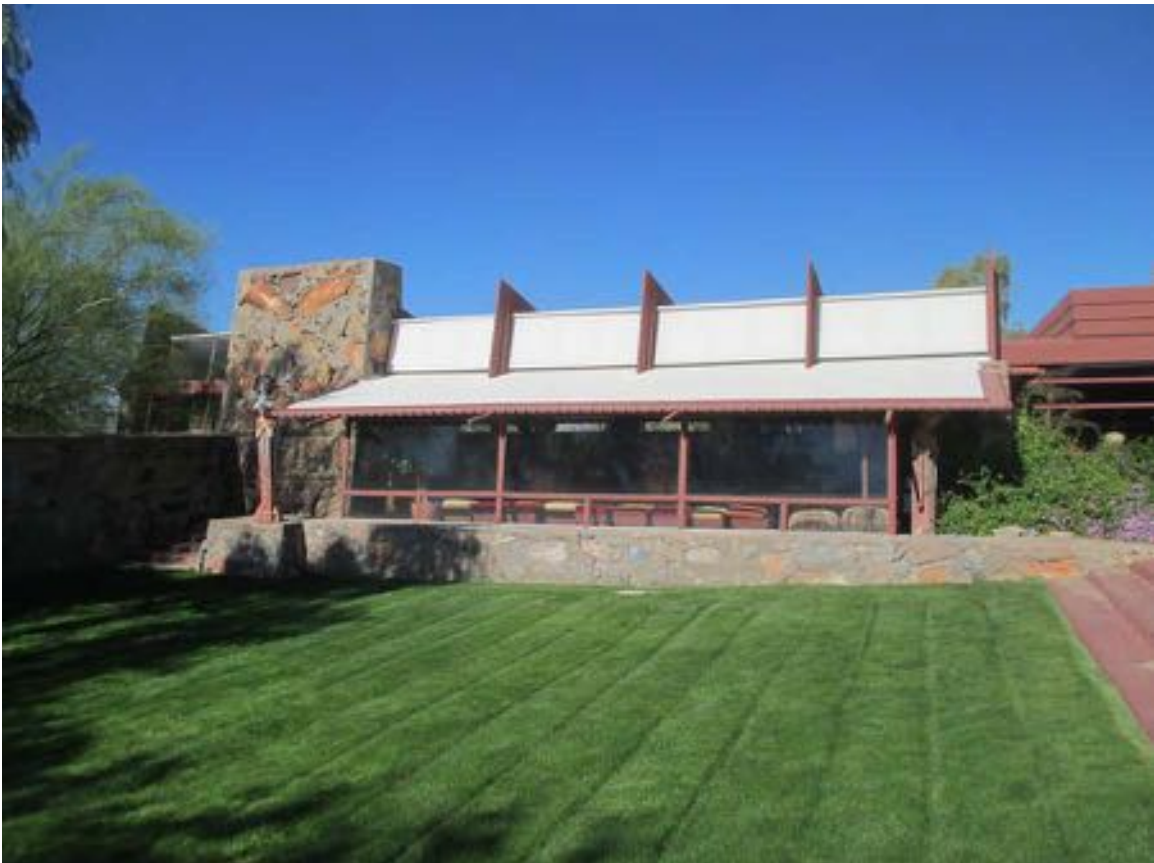
Figure 10-66 - Exterior of Garden Room looking northwest from garden, 2014 (Harboe Architects).
