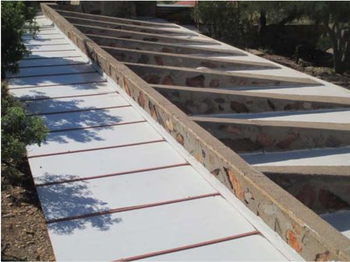
Figure 11-99 - Roof of Cabaret, 2014 (Harboe Architects).
