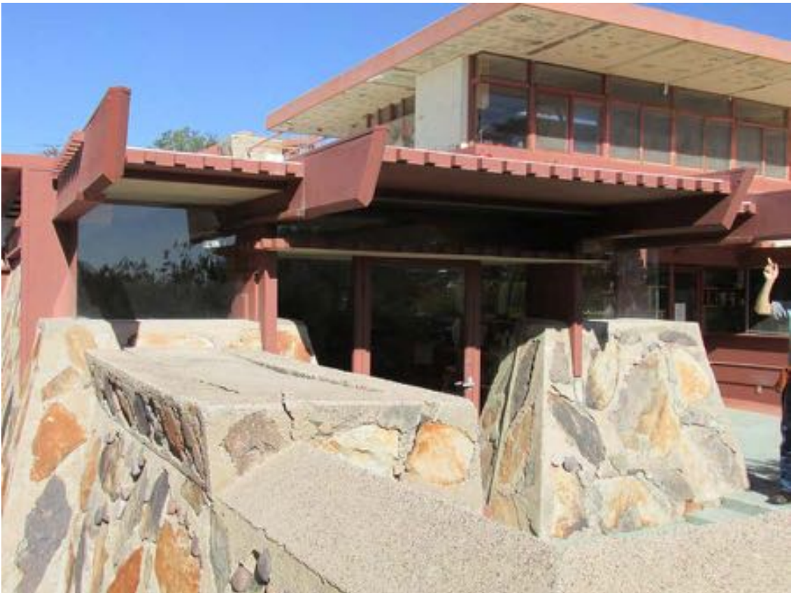
Figure 11-208 - Exterior of Dr. Joe Office, 2015 (Harboe Architects).
