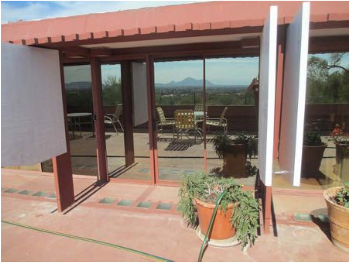
Figure 10-116 - Looking north at guest room with open wood flaps, 2014 (Harboe Architects).
