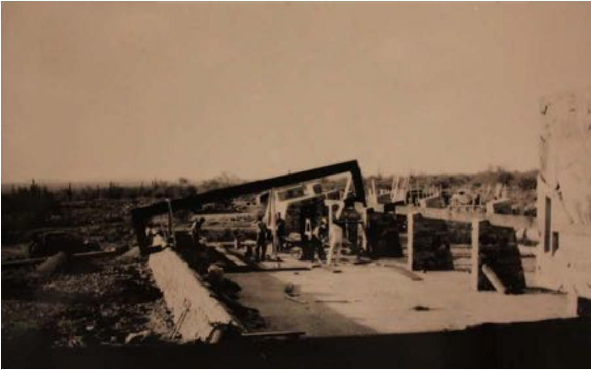
Figure 7-6 - Construction of the Drafting Studio, ca. 1938 (The Frank Lloyd Wright Foundation Archives, The Museum of Modern Art | Avery Architectural & Fine Arts Library, Columbia University, New York).
