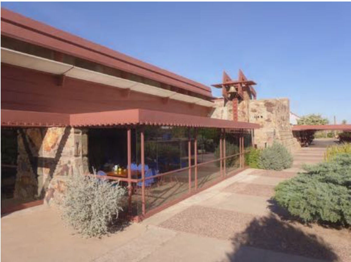
Figure 11-108 - Exterior of Dining Room looking west, 2014 (Harboe Architects).
