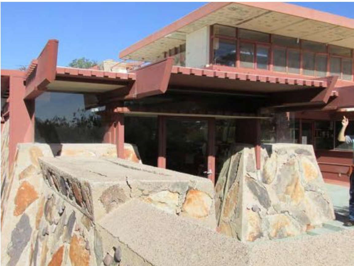
Figure 10-255 - Exterior of Dr. Joe Office, 2015 (Harboe Architects).
