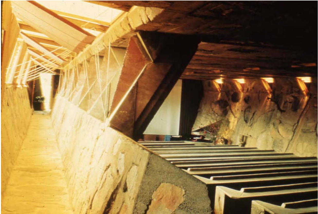
Figure 7-52 - Inside the Cabaret corridor with operable canvas panels, ca. 1952 (The Frank Lloyd Wright Foundation Archives, The Museum of Modern Art | Avery Architectural & Fine Arts Library, Columbia University, New York).
