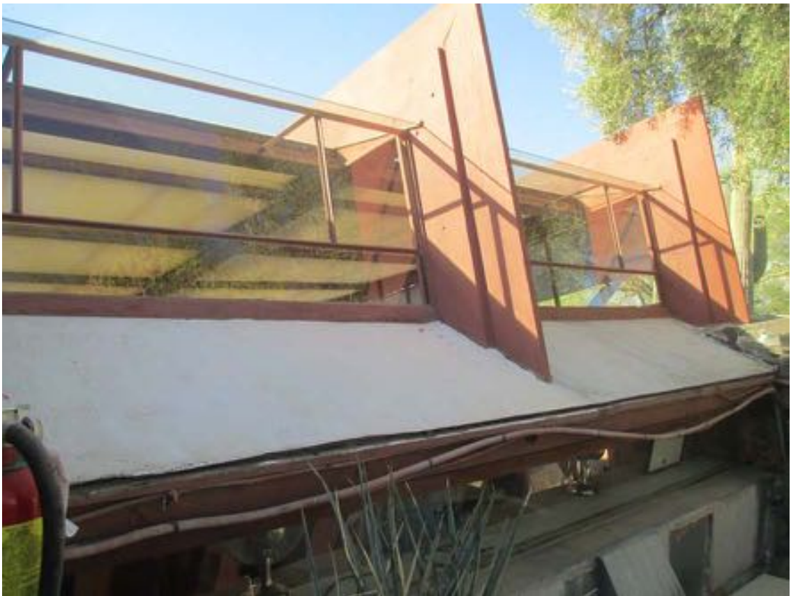
Figure 11-10 - North clerestory windows and roof on the office in 2014 (Harboe Architects).
