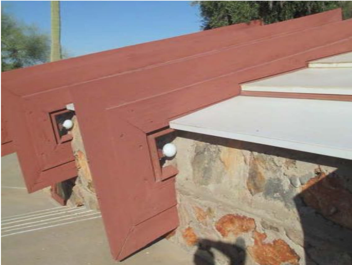
Figure 11-9 - Roof trusses on the office in 2014 (Harboe Architects).
