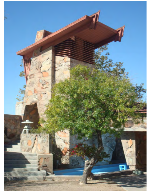
Figure 7-50 - Water Tower 2014 (Harboe Architects).
