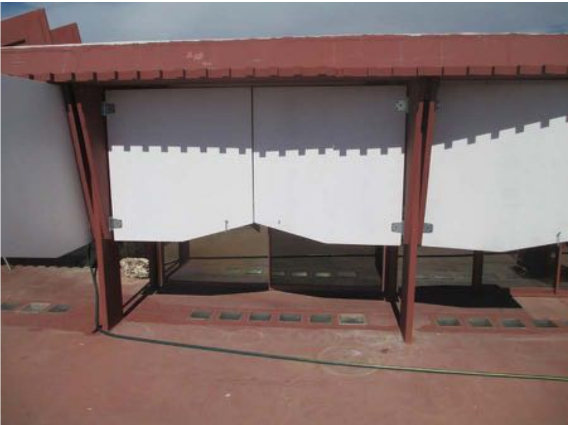
Figure 11-118 - Guest Deck looking north at guest room with closed wood flaps, 2014 (Harboe Architects).
