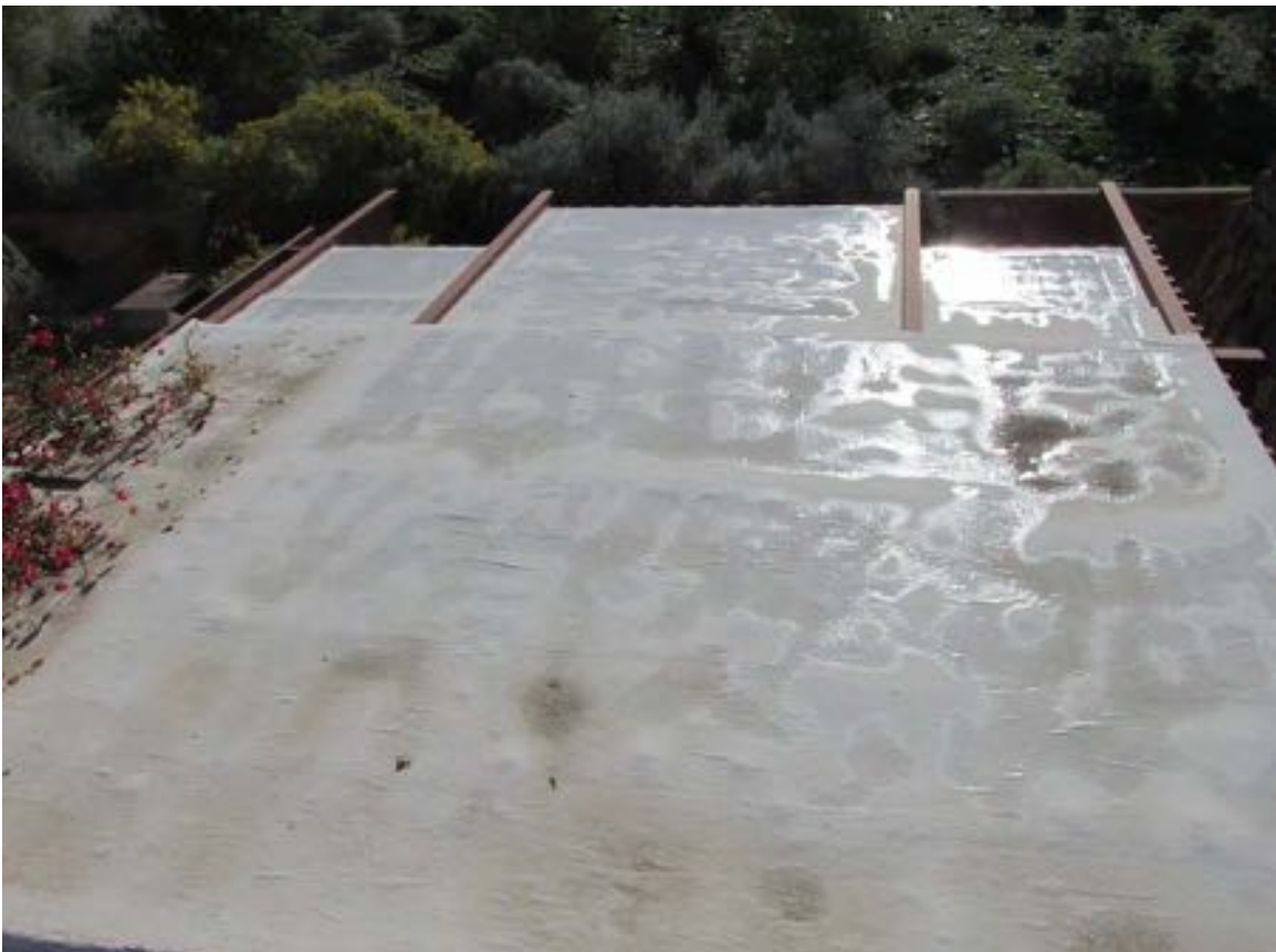
Figure 11-210 - Roof of Dr. Joe Office, 2015 (Harboe Architects).
