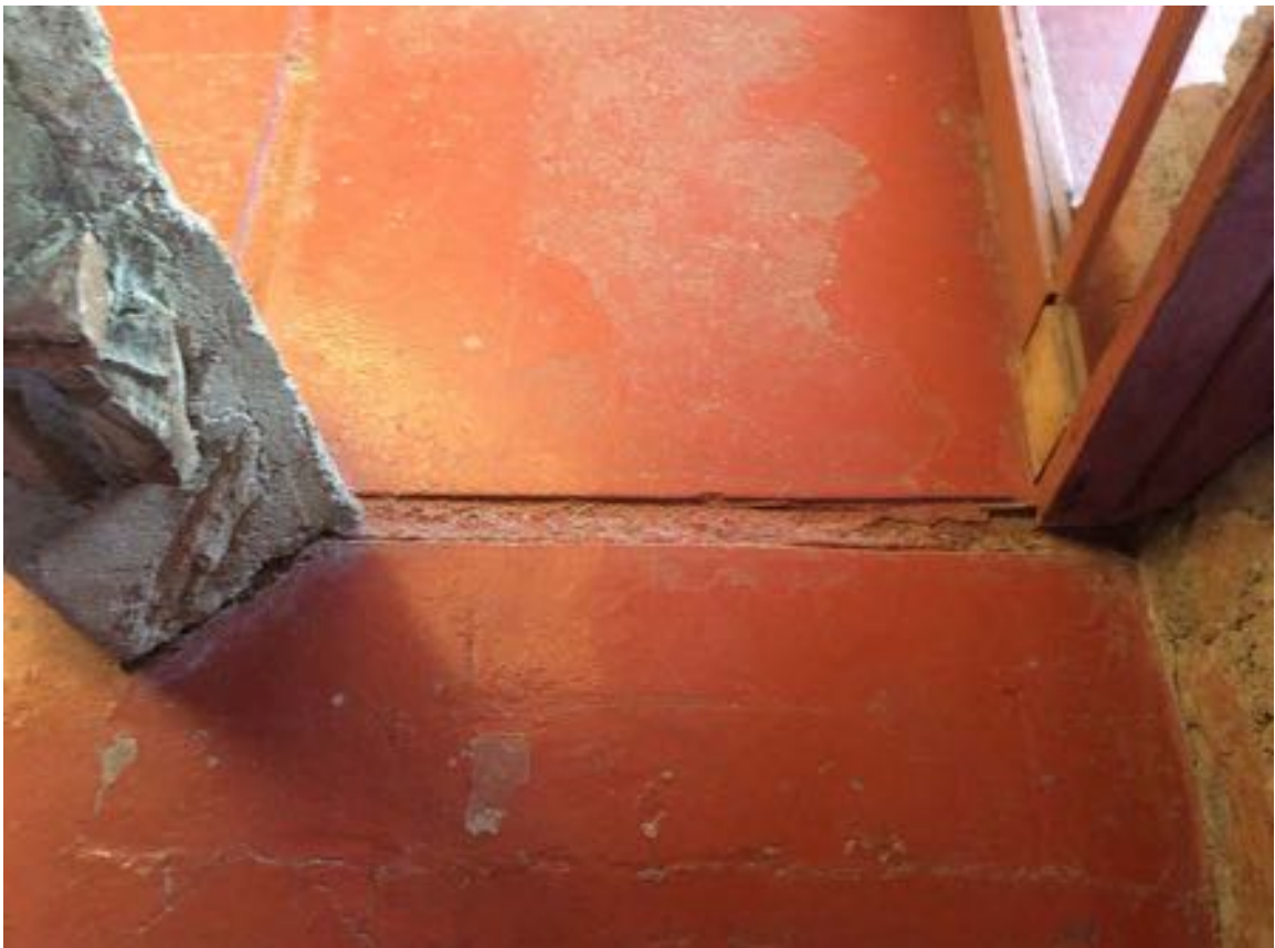
Figure 10-46 - Board room floor, 2014 (Harboe Architects).
