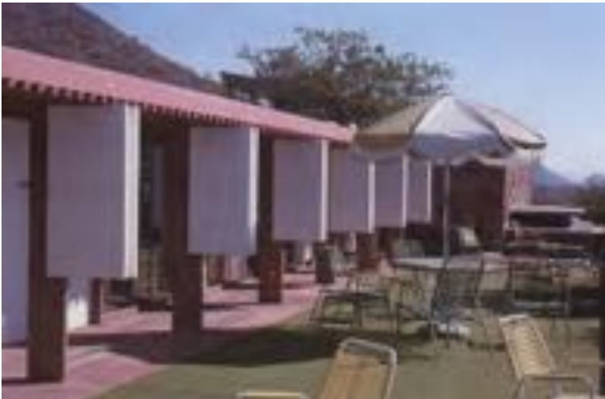
Figure 7-64 - Guest Deck, ca. 1975 (The Frank Lloyd Wright Foundation Archives, The Museum of Modern Art | Avery Architectural & Fine Arts Library, Columbia University, New York).
