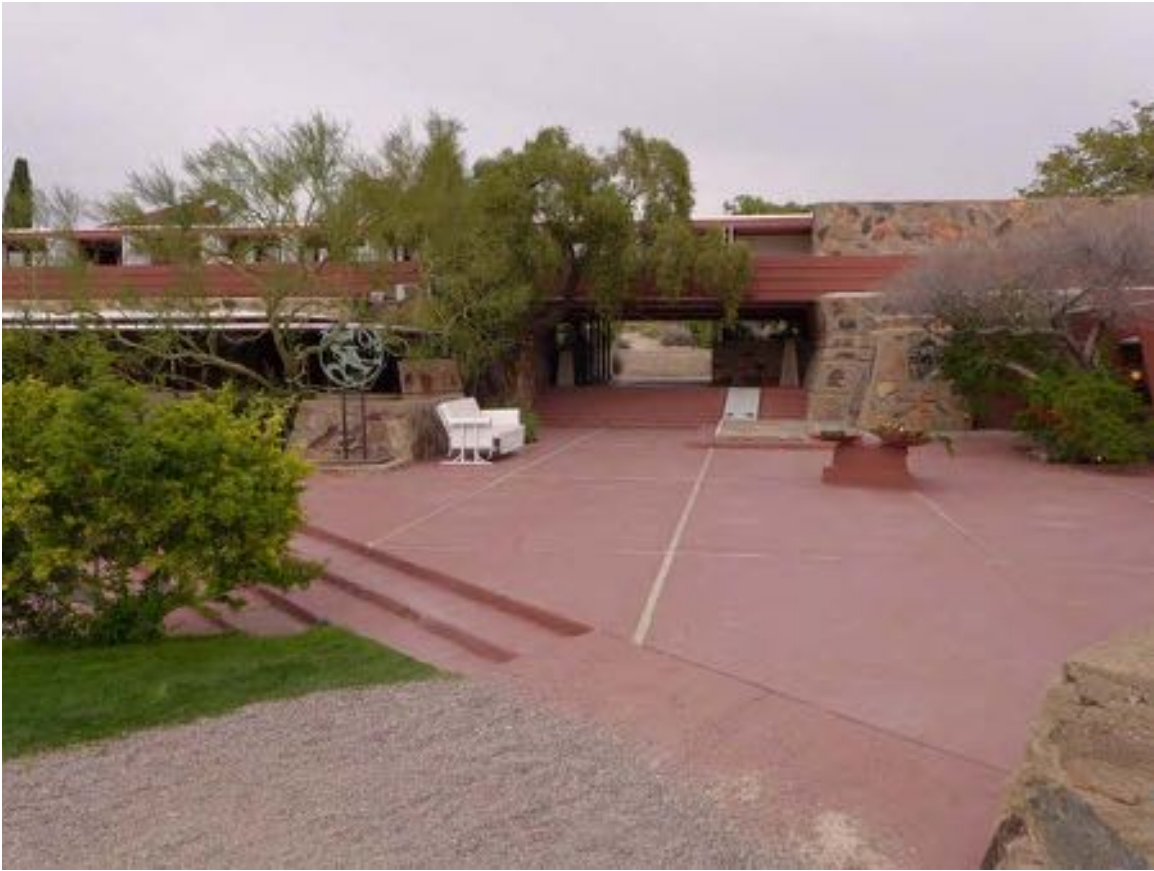
Figure 11-251 - Sunset Terrace, 2014 (Harboe Architects).
