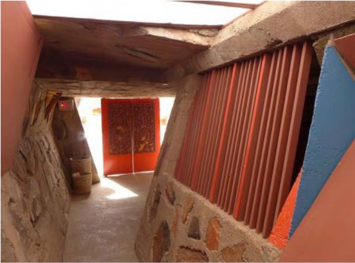
Figure 10-95 - Cabaret corridor looking south at entry doors, 2014 (Harboe Architects).
