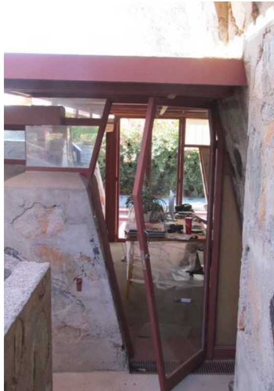
Figure 10-262 - Door to Dr. Joe Office from exterior, 2015 (Harboe Architects).
