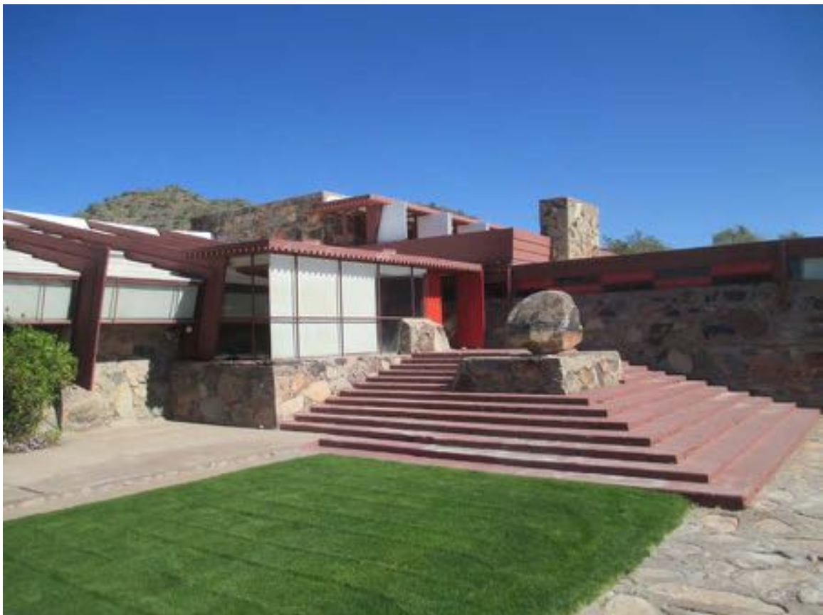
Figure 11-21 - Solarium and terrace on southeast side of Drafting Studio, 2014 (Harboe Architects).
