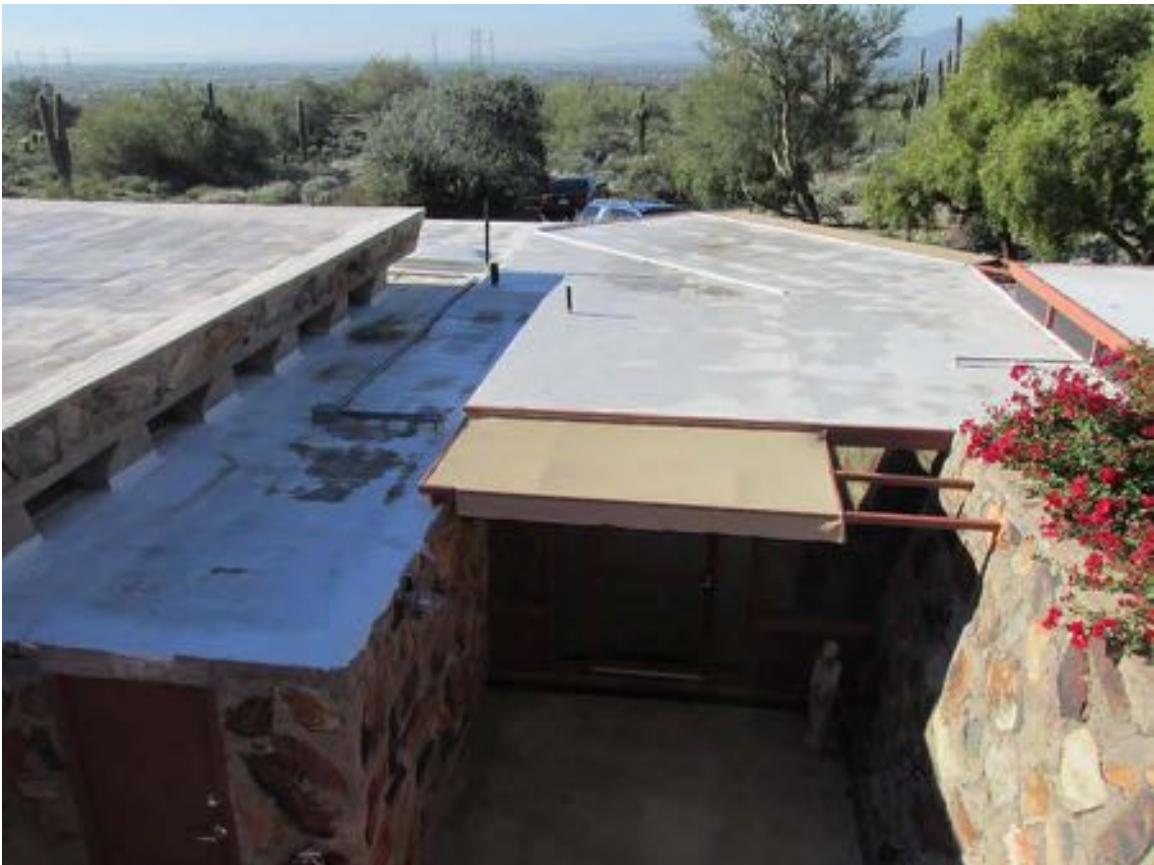
Figure 10-277 - Roof of Carney Office, 2015 (Harboe Architects).
