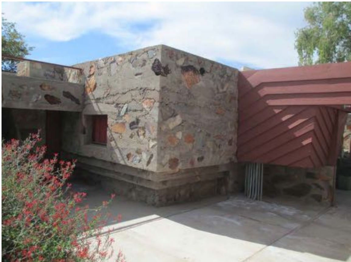
Figure 10-50 - Exterior of Kiva looking west, 2014 (Harboe Architects).
