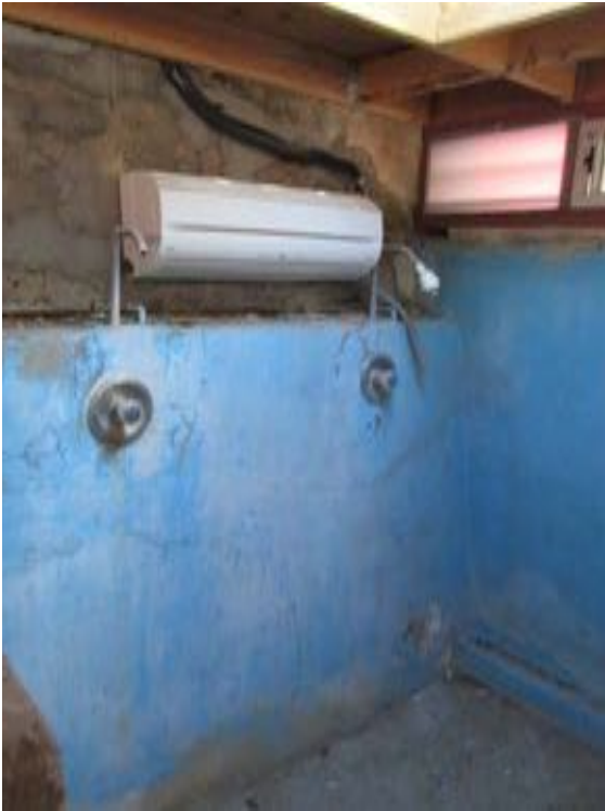
Figure 10-128 - Shower area in Old Men's Locker Room, 2015 (Harboe Architects).
