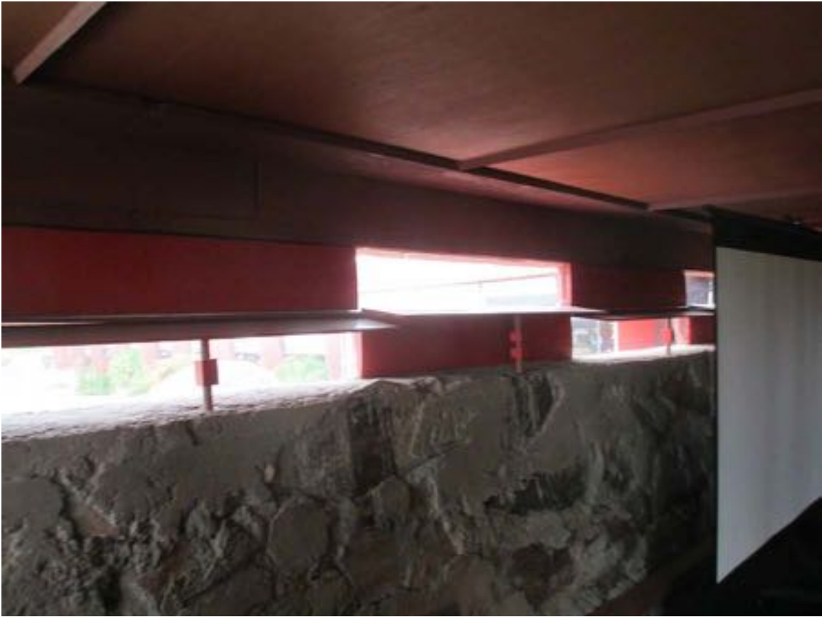
Figure 11-47 - Windows on northwest wall of Original Dining Room, 2014 (Harboe Architects).
