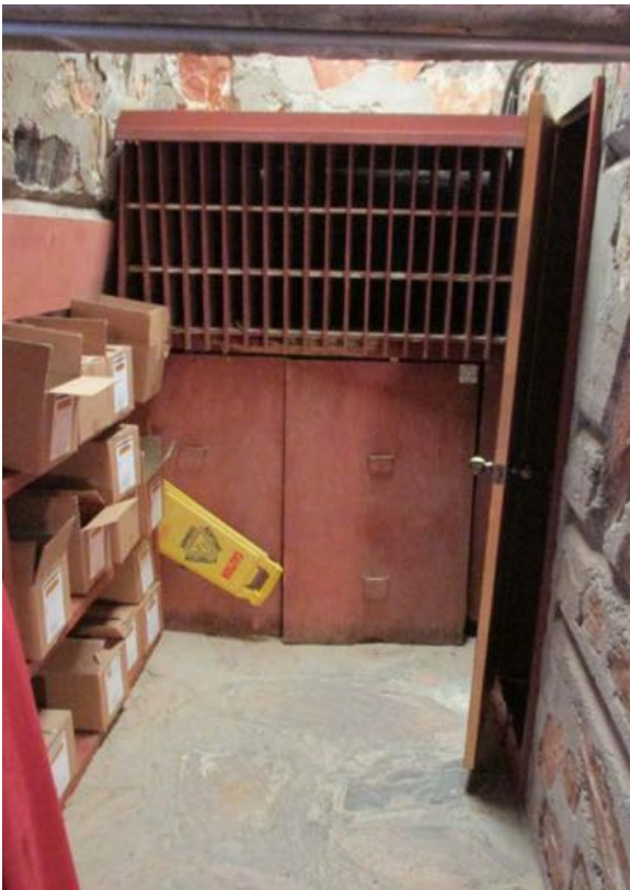
Figure 10-100 - Mailbox area outside of the men's restroom, 2015 (Harboe Architects).
