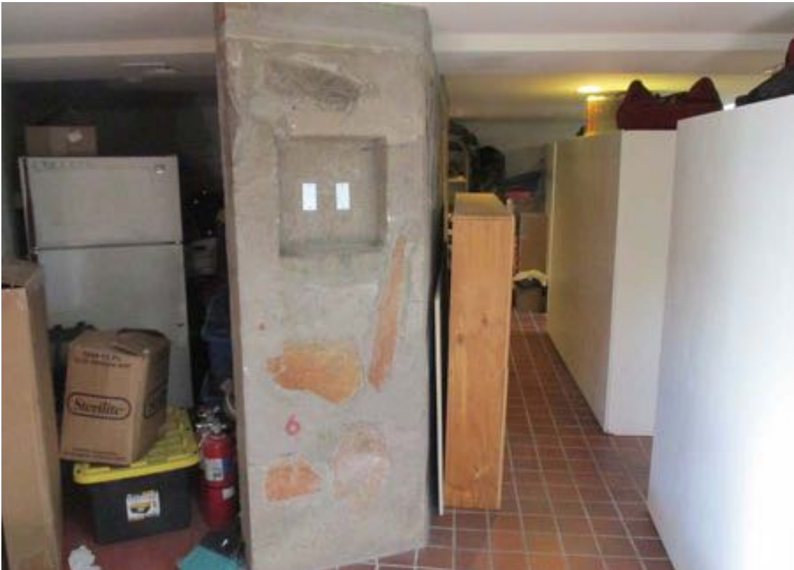
Figure 11-142 - Storage area inside Men's Locker Room, 2015 (Harboe Architects).
