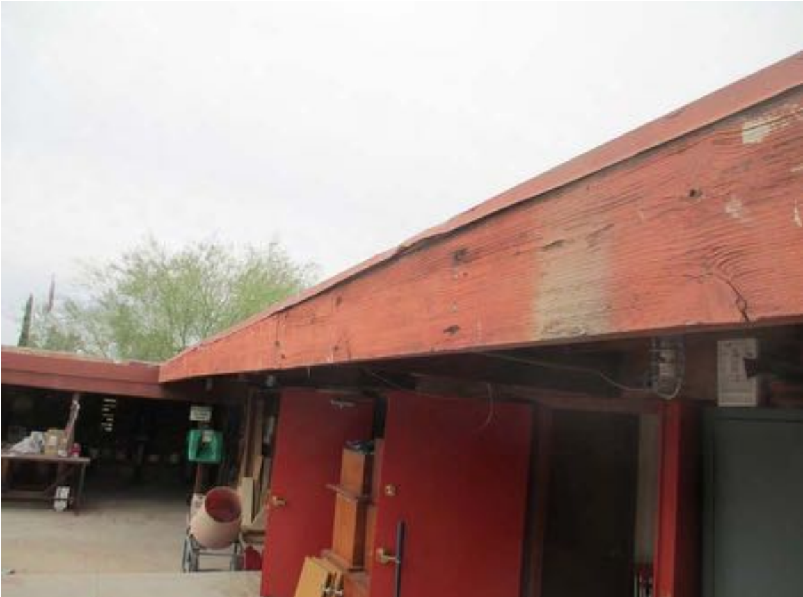
Figure 10-140 - View of Shops showing wood fascia at eaves, 2014 (Harboe Architects).
