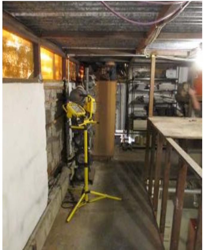
Figure 10-191 - Catwalk, 2015 (Harboe Architects).
