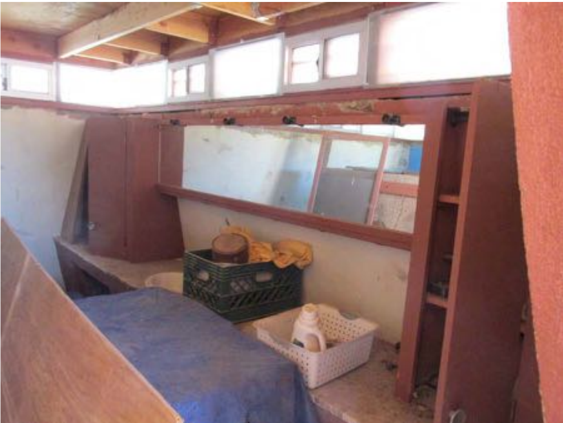
Figure 10-127 - Sink area in Old Men's Locker Room, 2015 (Harboe Architects).
