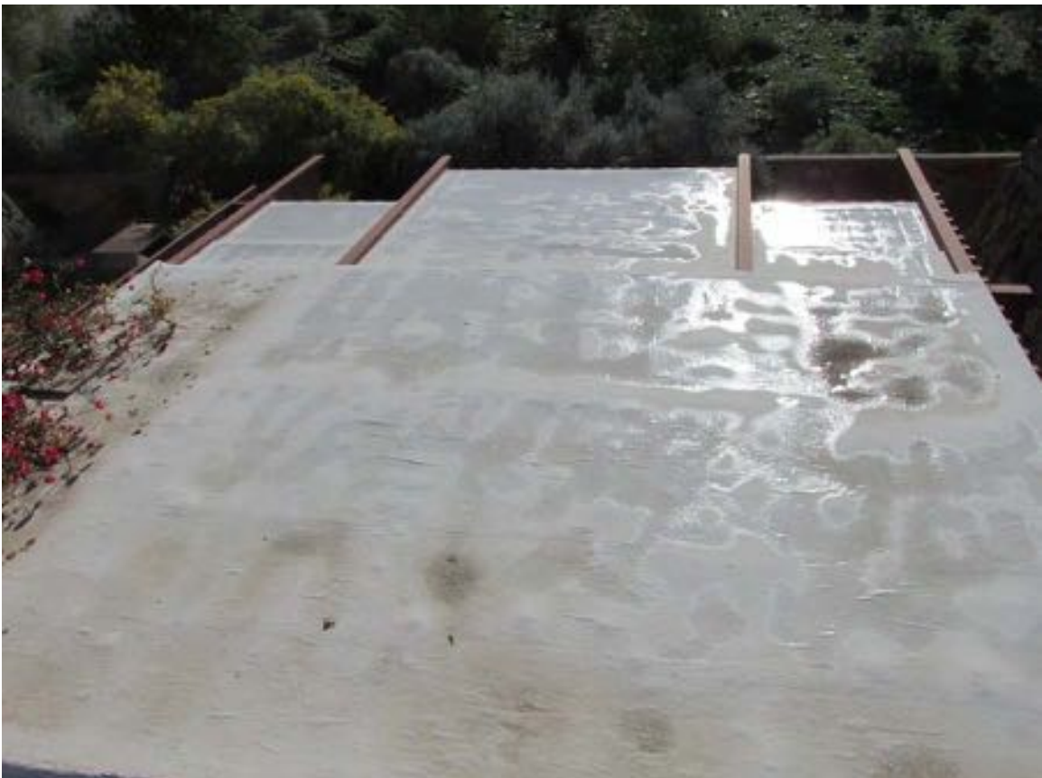
Figure 10-257 - Roof of Dr. Joe Office, 2015 (Harboe Architects).
