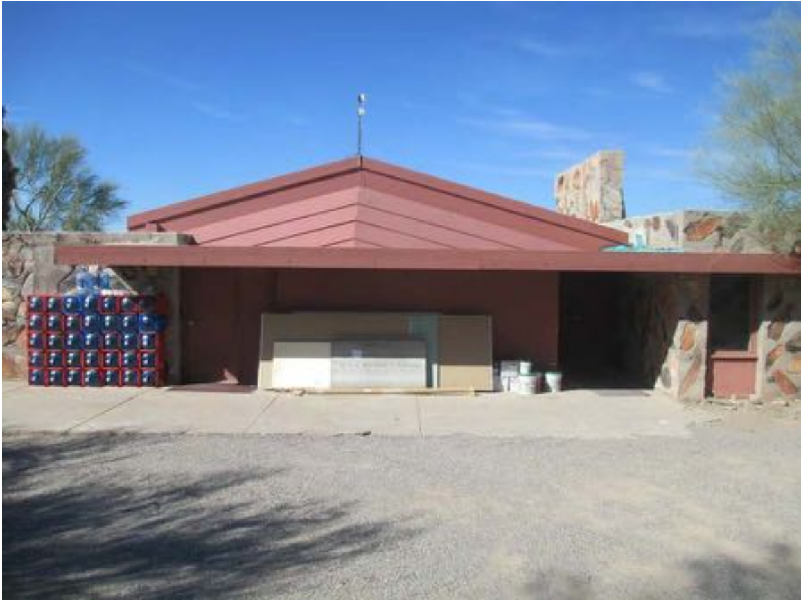
Figure 11-162 - East side of the Pavilion, 2014 (Harboe Architects).
