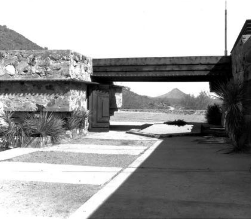
Figure 7-102 - Original Kiva Bridge, ca. 1942 (The Frank Lloyd Wright Foundation Archives, The Museum of Modern Art | Avery Architectural & Fine Arts Library, Columbia University, New York).
