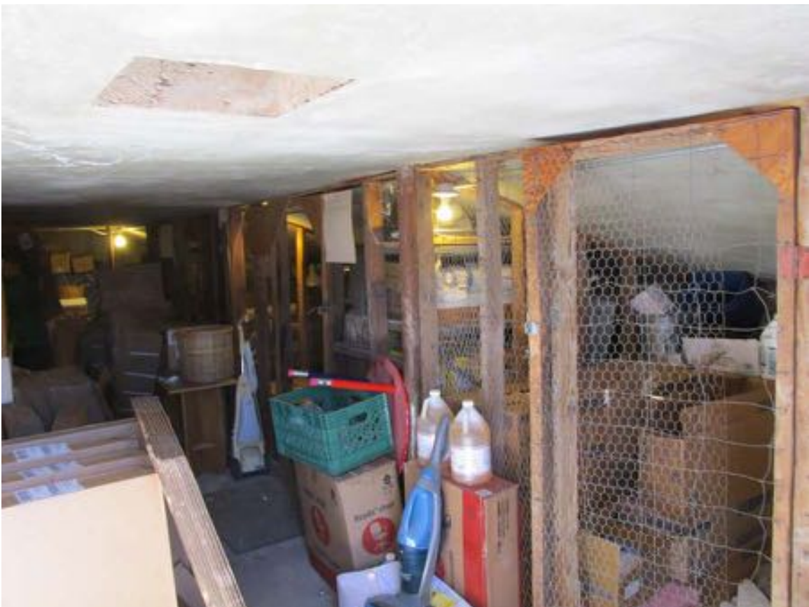
Figure 10-143 - Inside the Root Cellar, 2015 (Harboe Architects).
