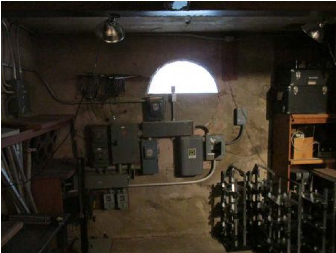
Figure 10-103 - Cabaret projection room, 2015 (Harboe Architects).
