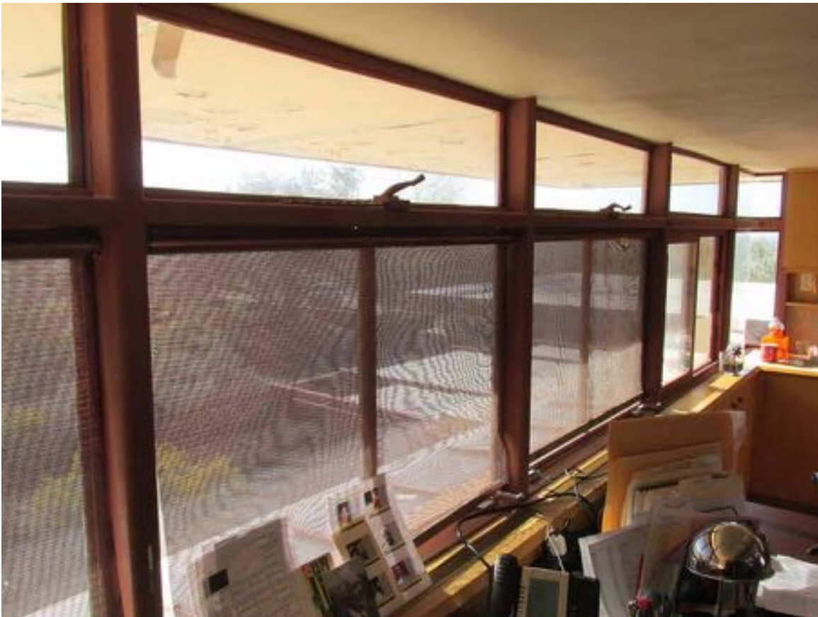
Figure 10-295 - Windows along east wall of Tower Office, 2015 (Harboe Architects).
