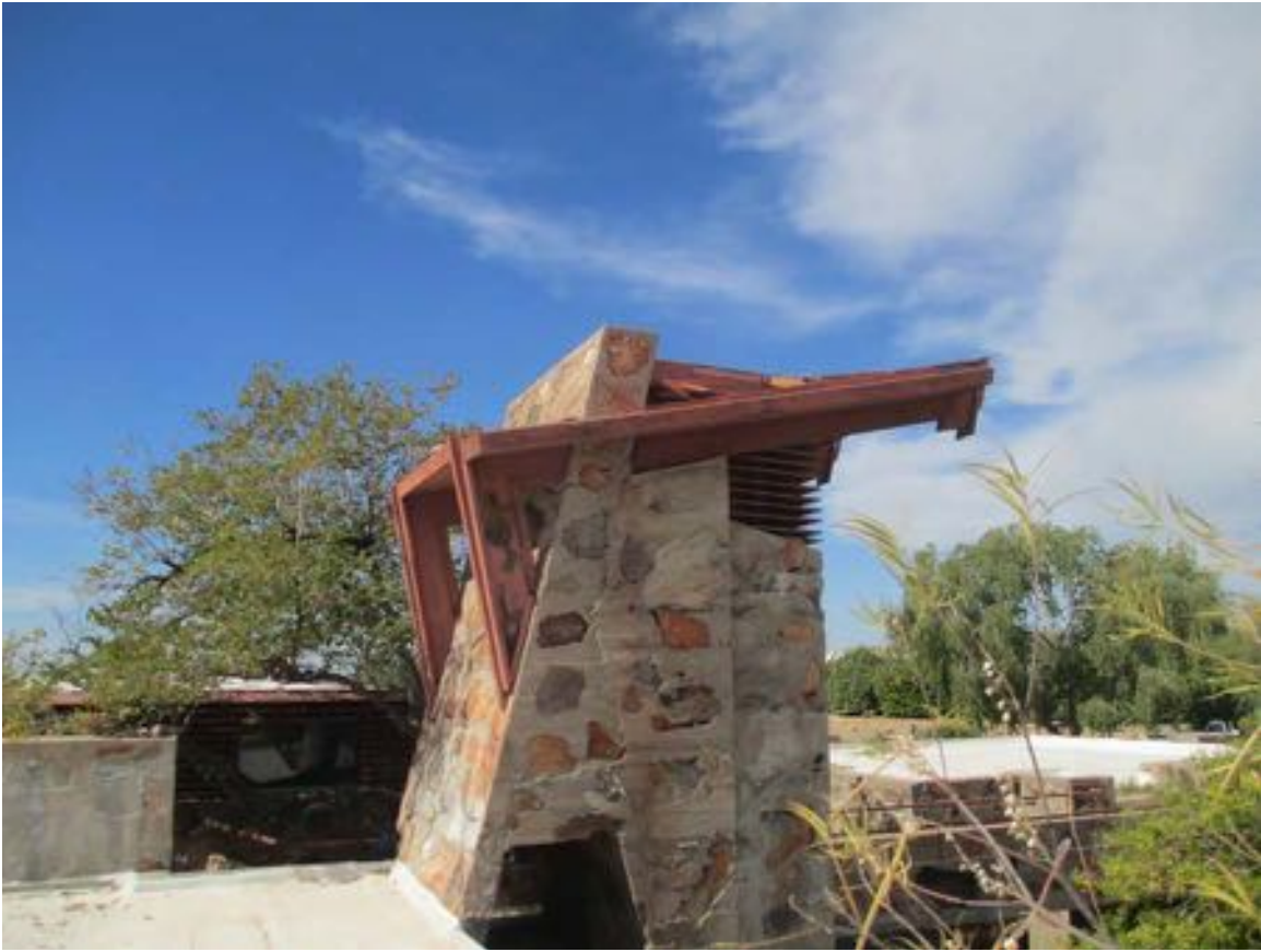
Figure 11-90 - Water Tower, 2014 (Harboe Architects).
