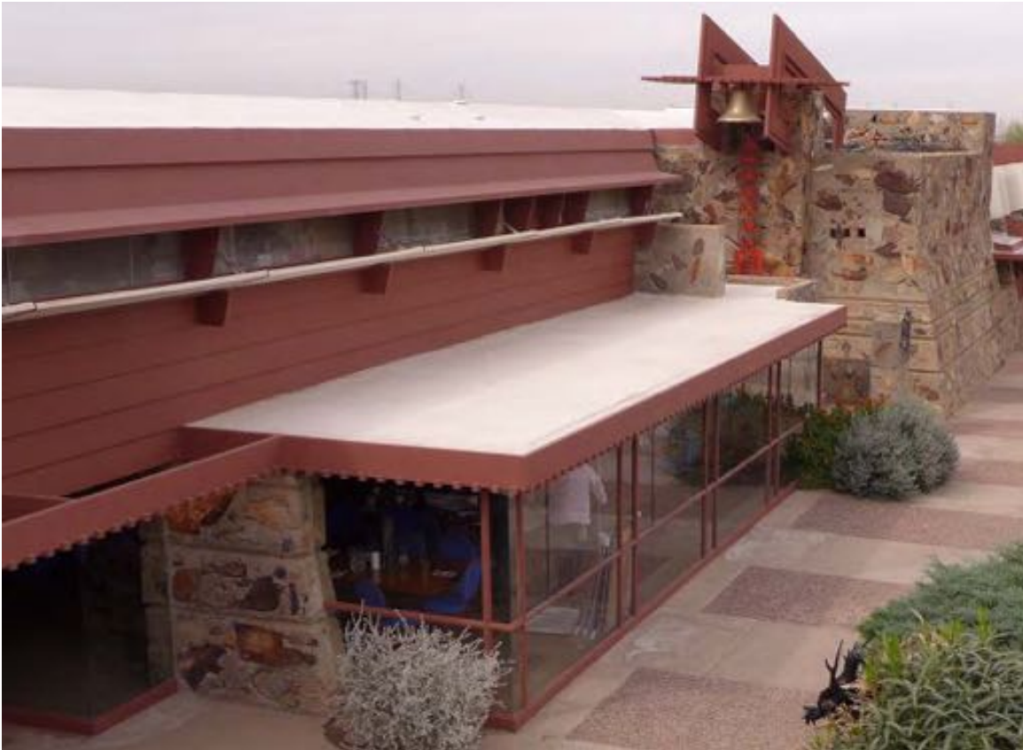
Figure 10-106 - View of Dining Room from Kiva roof, 2014 (Harboe Architects).
