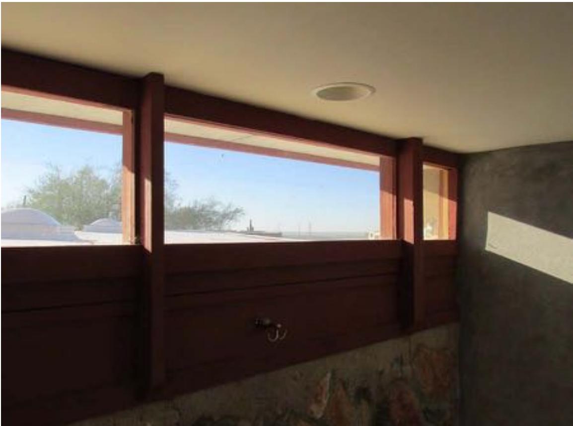
Figure 10-149 - Windows above sinks inside Men's Locker Room, 2015 (Harboe Architects).
