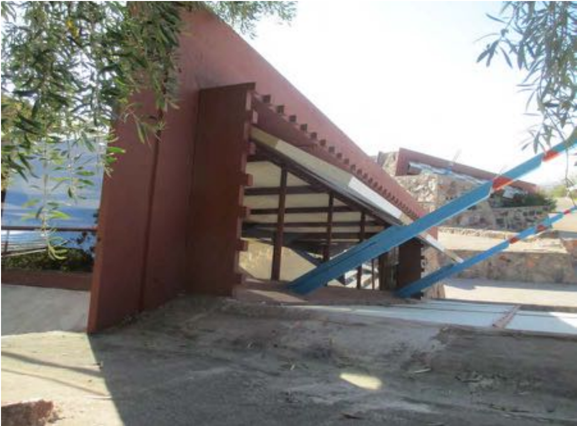
Figure 10-7 - Sunshade and supports on the office in 2014 (Harboe Architects).
