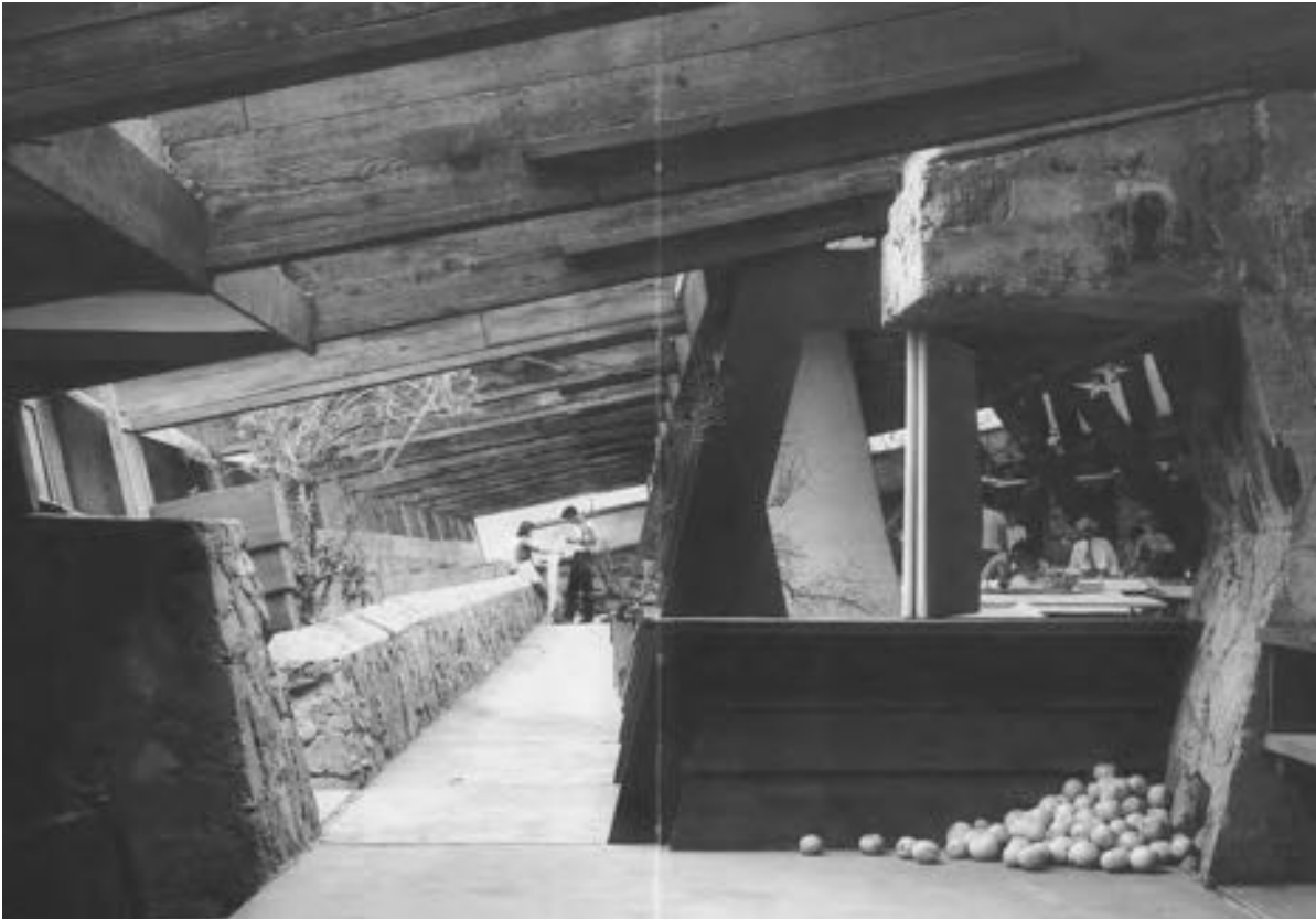
Figure 7-11 - Walkway on south side of the Drafting Studio, 1946 (Ezra Stoller)
