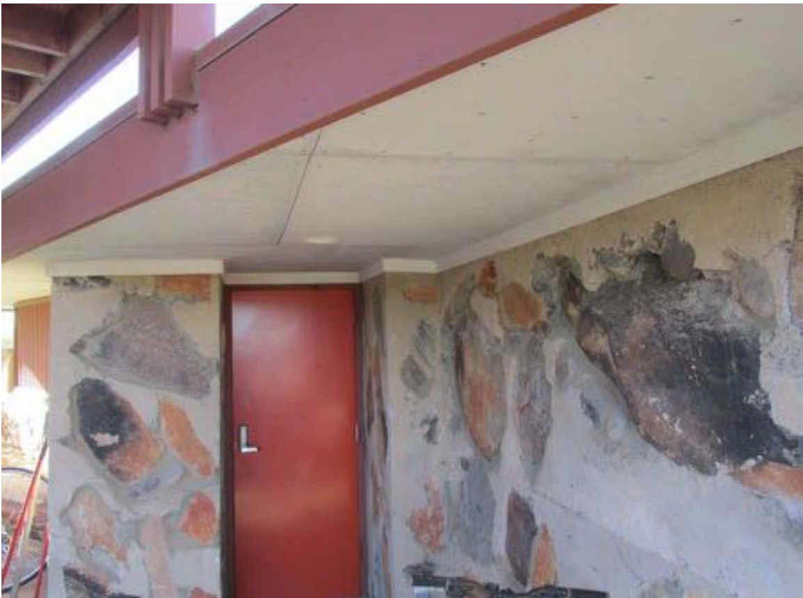
Figure 11-140 - Soffit on northeast side of Men's Locker Room, 2015 (Harboe Architects).
