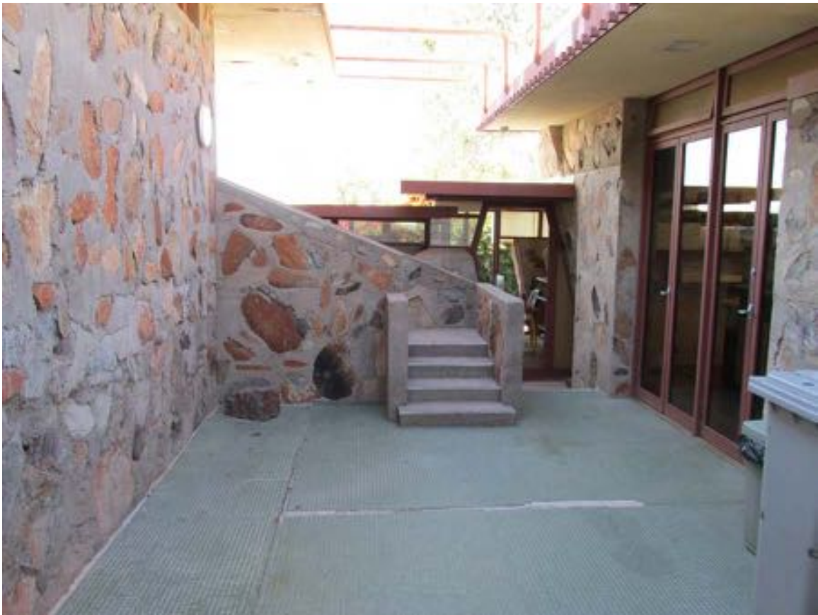
Figure 11-190 - Courtyard outside the Finance Office, 2015 (Harboe Architects).
