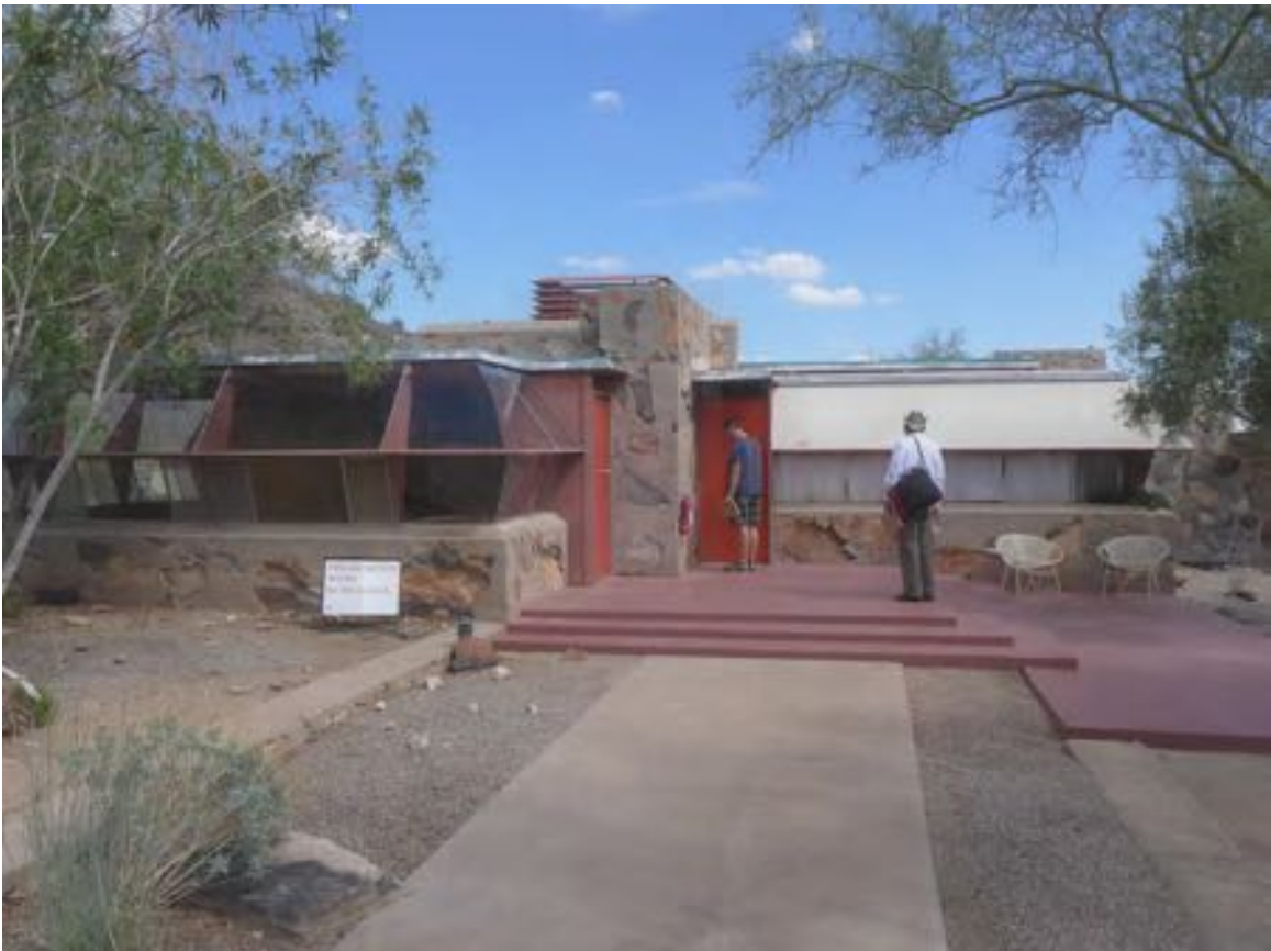
Figure 10-167 - Looking northeast at Sun Cottage, 2014 (Harboe Architects).
