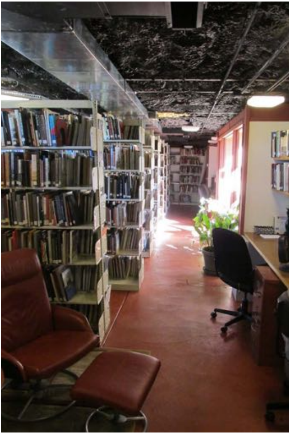
Figure 11-174 - Inside library, 2015 (Harboe Architects).
