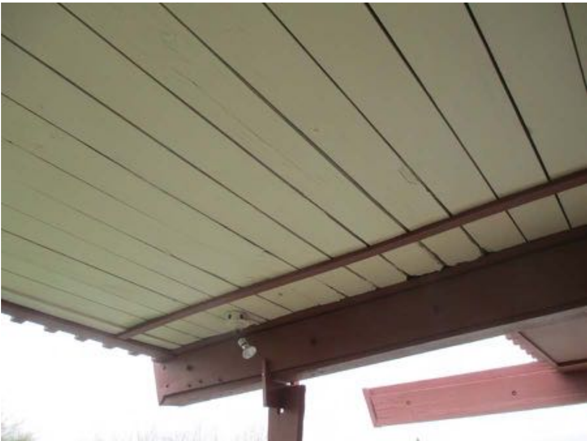
Figure 10-40 - Underside of wood deck, 2014 (Harboe Architects).
