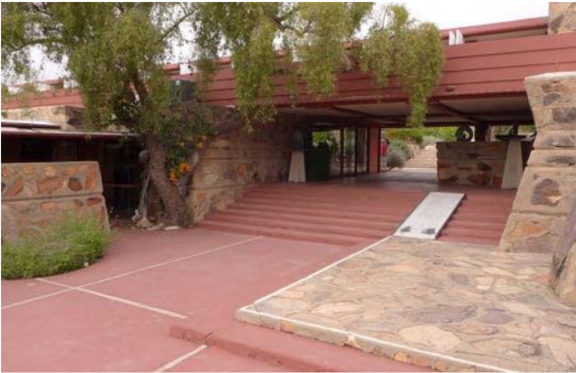
Figure 11-252 - Sunset Terrace, 2014 (Harboe Architects).
