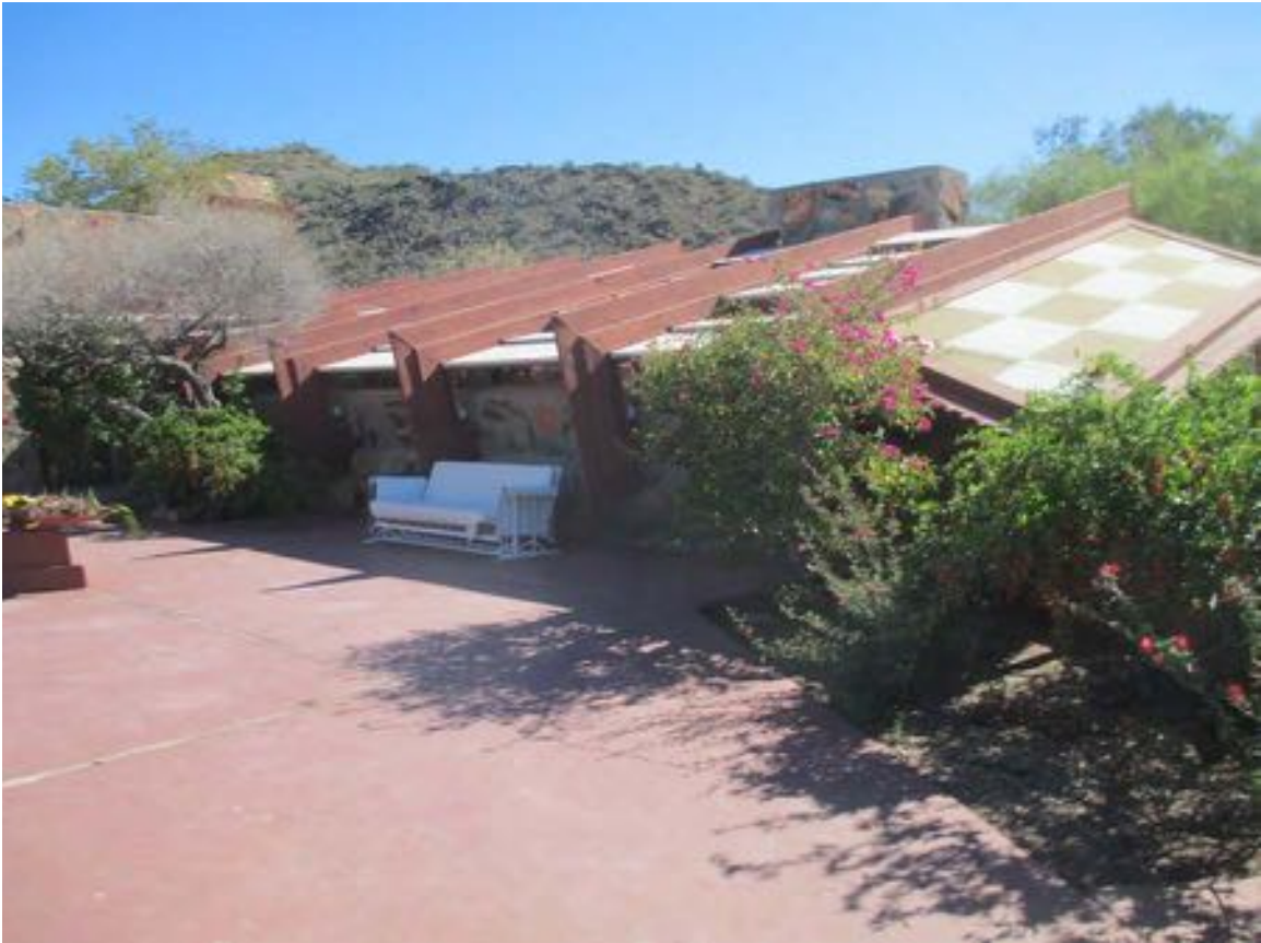
Figure 10-65 - Exterior of Garden Room looking east, 2014 (Harboe Architects).
