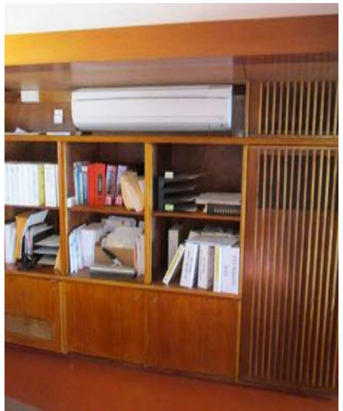
Figure 10-251 - Built-in wood shelves in Dekoven Hill office, 2015 (Harboe Architects).
