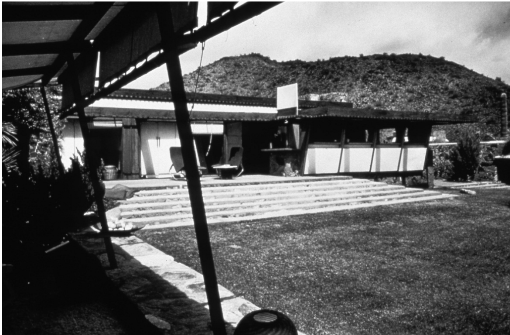
Figure 7-43 - View of the Wrights' Living Quarters from the Garden Room porch, ca. 1945 (The Frank Lloyd Wright Foundation Archives, The Museum of Modern Art | Avery Architectural & Fine Arts Library, Columbia University, New York).
