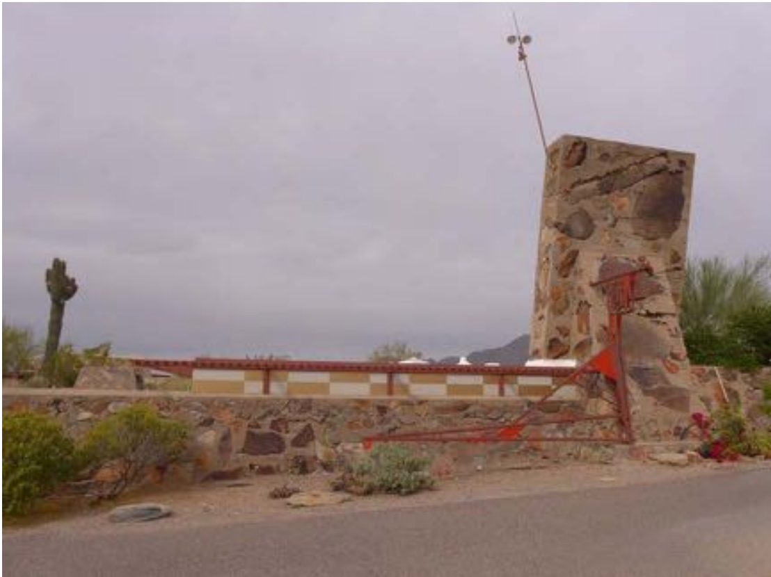
Figure 11-132 - View of Shops and Light Tower looking north, 2014 (Harboe Architects).
