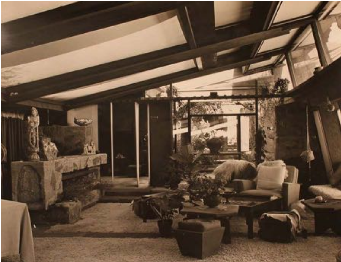
Figure 6-26 - Garden Room looking north after glass installed at clerestory and north wall, ca. 1948 (The Frank Lloyd Wright Foundation Archives, The Museum of Modern Art | Avery Architectural & Fine Arts Library, Columbia University, New York).
