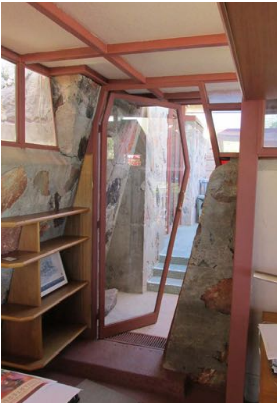
Figure 10-261 - Door to Dr. Joe Office from interior, 2015 (Harboe Architects).
