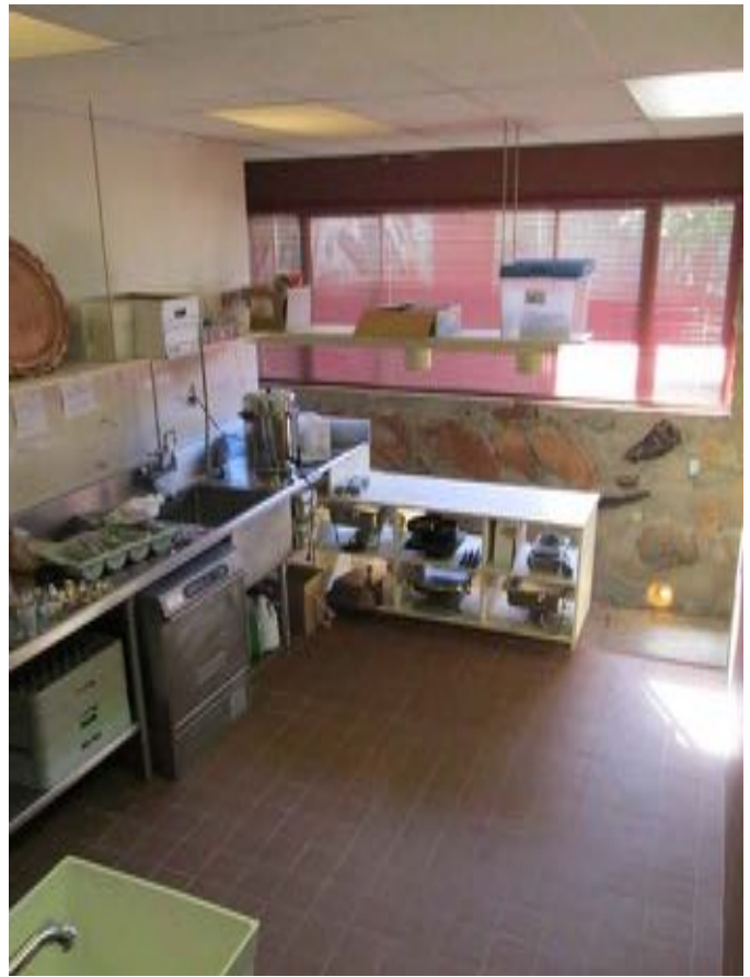
Figure 10-189 - Pavilion kitchen, 2015 (Harboe Architects).
