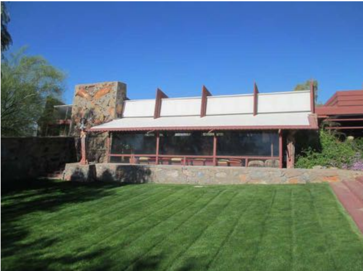
Figure 11-77 - Exterior of Garden Room looking northwest from garden, 2014 (Harboe Architects).
