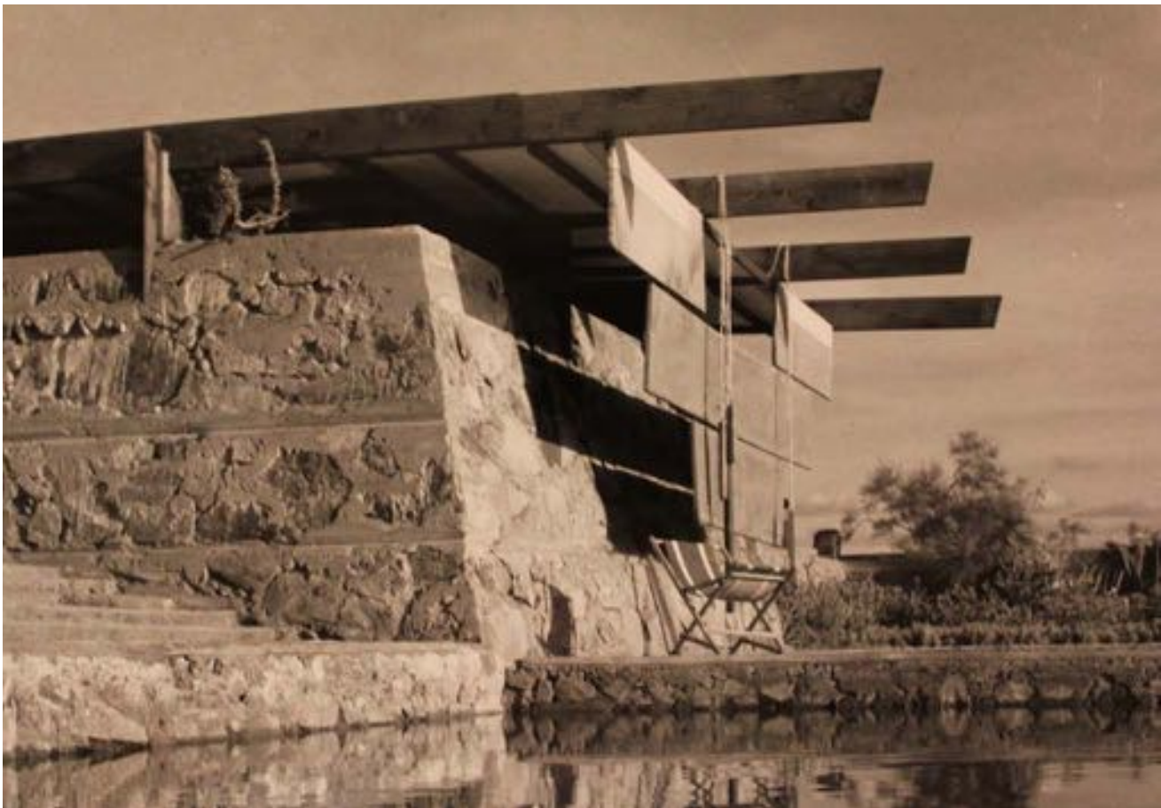
Figure 6-16 - Exterior of Original Dining Room, ca. 1939 (The Frank Lloyd Wright Foundation Archives, The Museum of Modern Art | Avery Architectural & Fine Arts Library, Columbia University, New York).
