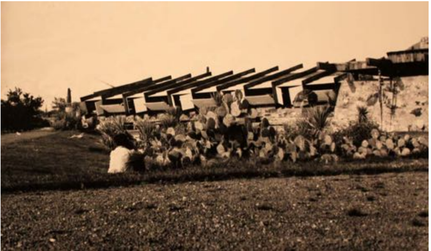
Figure 8-6 - Exterior of the Drafting Studio and Original Dining Room, ca. 1940 (The Frank Lloyd Wright Foundation Archives, The Museum of Modern Art | Avery Architectural & Fine Arts Library, Columbia University, New York).
