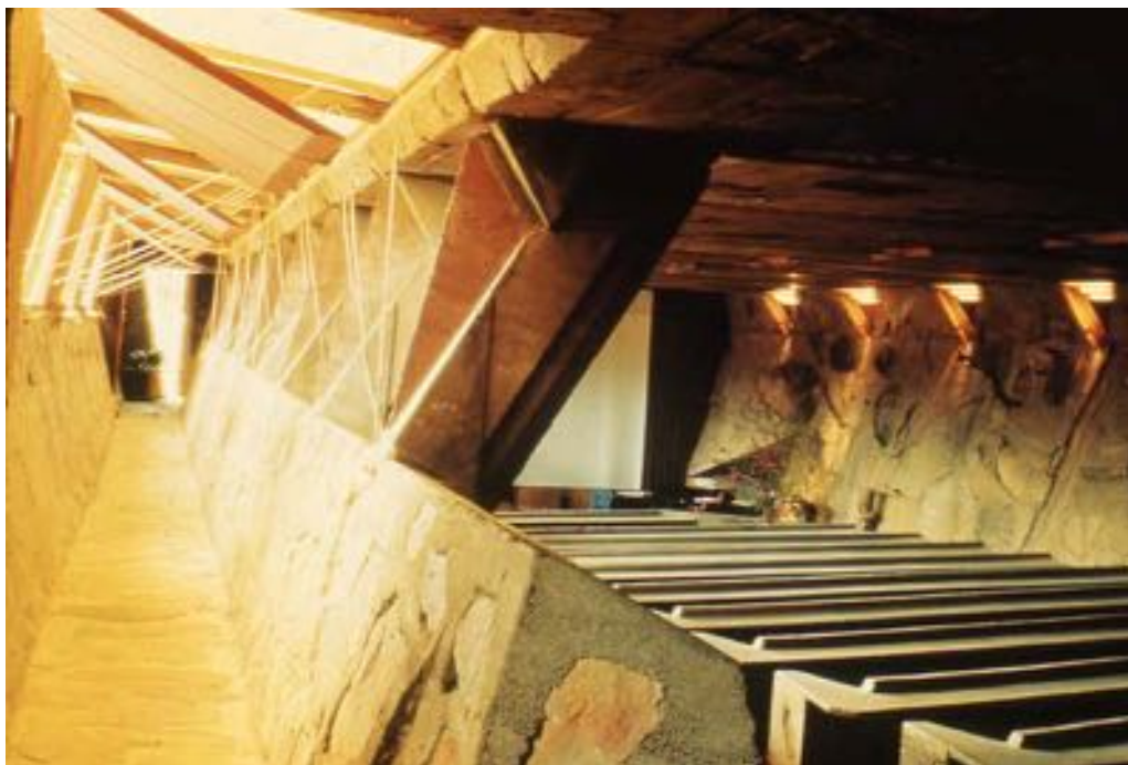
Figure 11-94 - Interior of Cabaret looking south at operable canvas flaps, ca. 1955 (The Frank Lloyd Wright Foundation Archives, The Museum of Modern Art | Avery Architectural & Fine Arts Library, Columbia University, New York).
