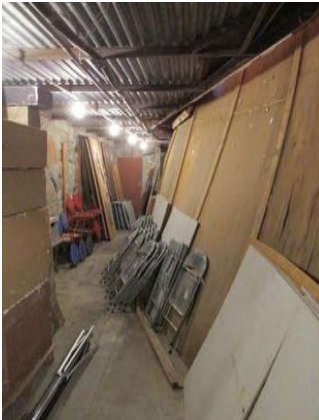
Figure 10-190 - Back of stage storage room, 2015 (Harboe Architects).
