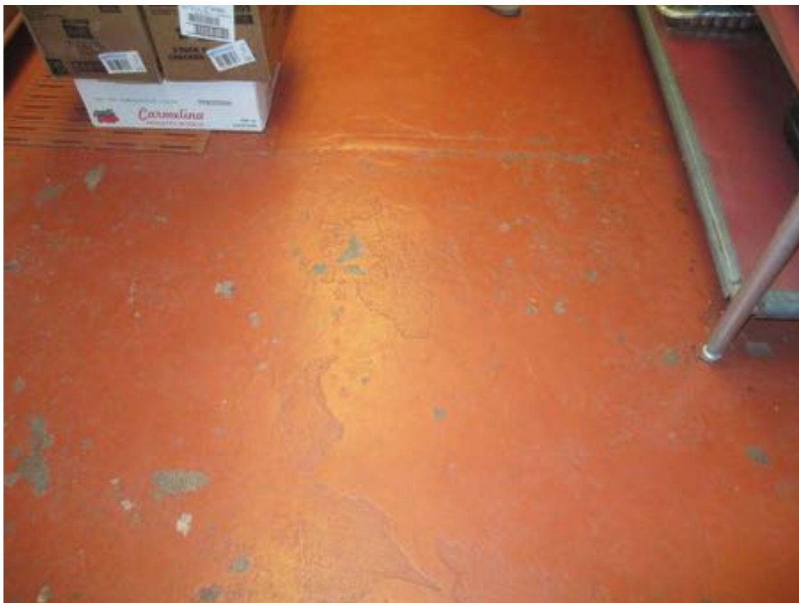
Figure 10-32 - Kitchen floor, 2014 (Harboe Architects).
