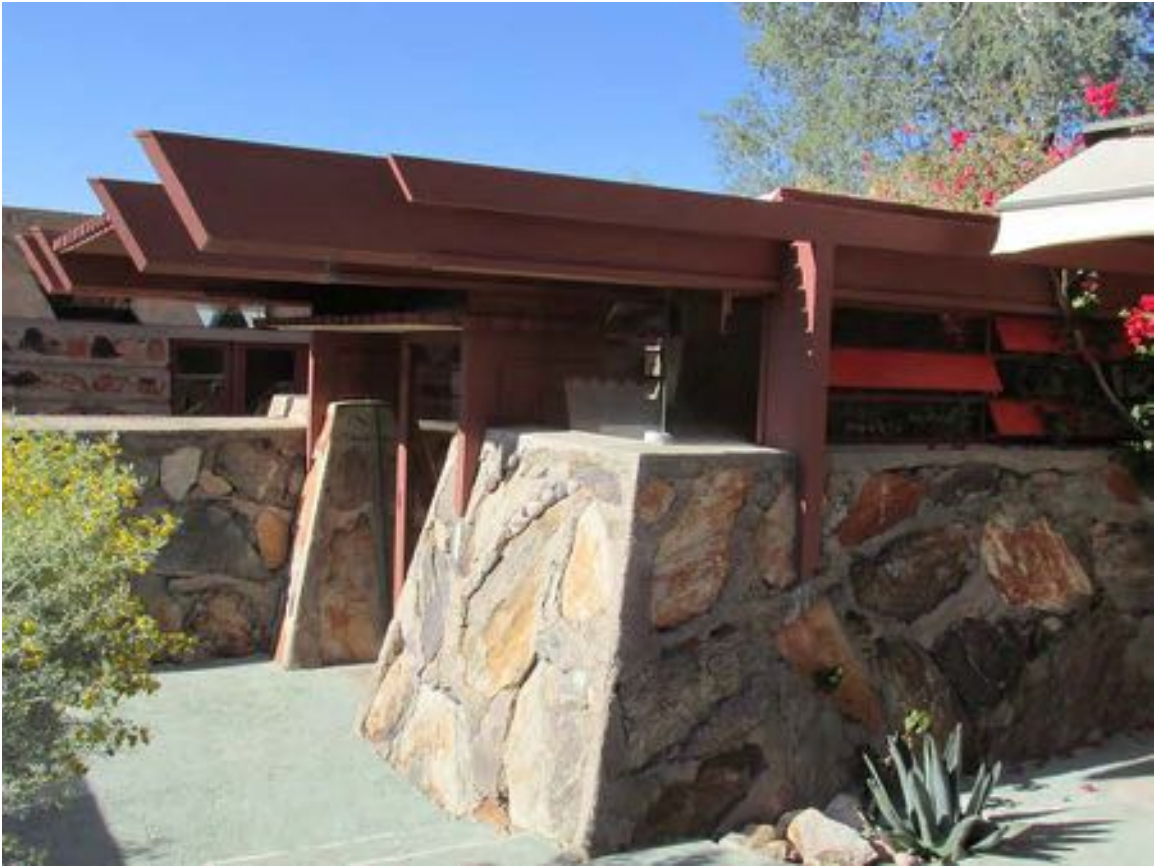
Figure 10-254 - Exterior of Dr. Joe Office, 2015 (Harboe Architects).
