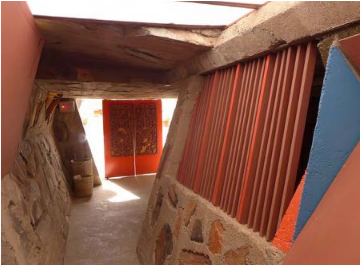
Figure 11-102 - Cabaret corridor looking south at entry doors, 2014 (Harboe Architects).
