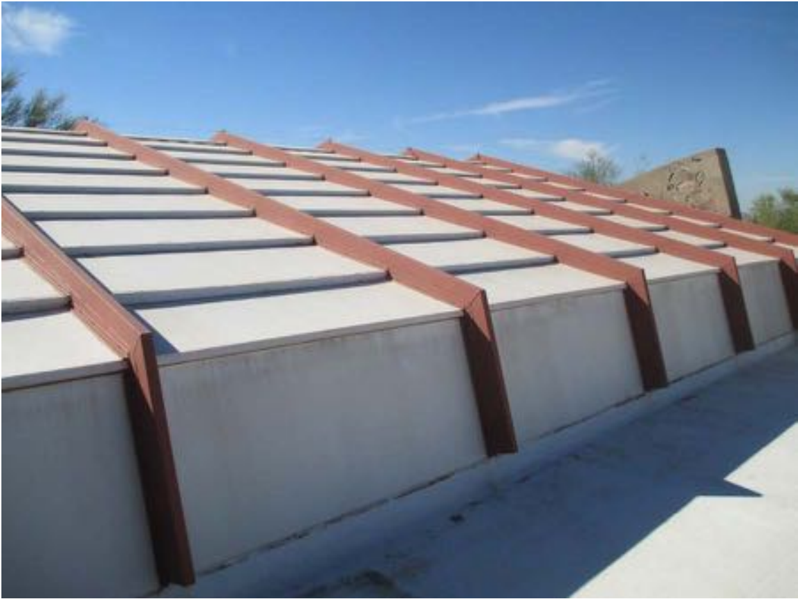
Figure 11-160 - Pavilion roof, 2014 (Harboe Architects).
