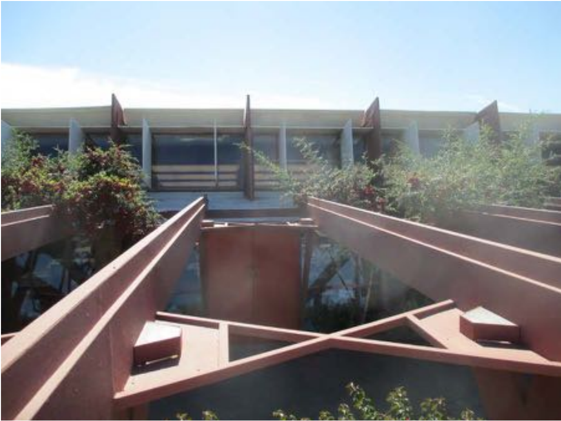
Figure 10-19- Pergola on north side of Drafting Studio, 2014 (Harboe Architects).
