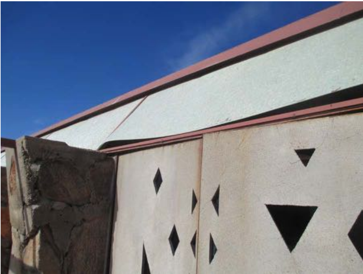
Figure 10-209 - Concrete panels and fiberglass panels above, 2014 (Harboe Architects).
