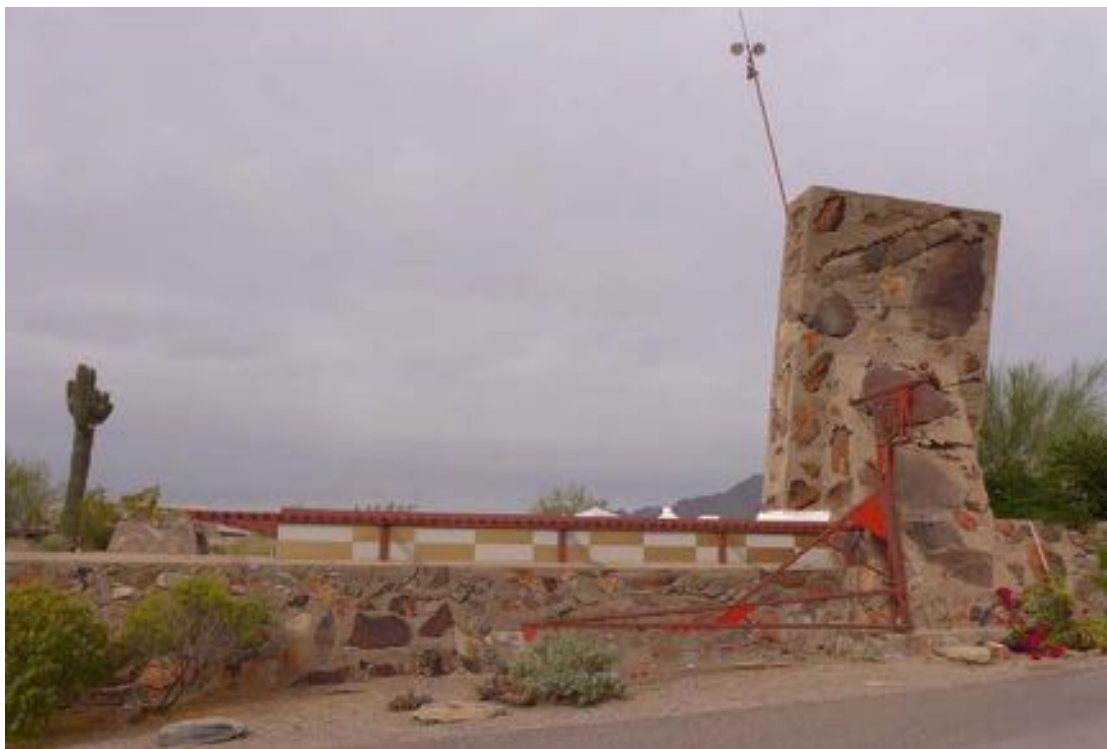
Figure 10-137 - View of Shops and Light Tower looking north, 2014 (Harboe Architects).
