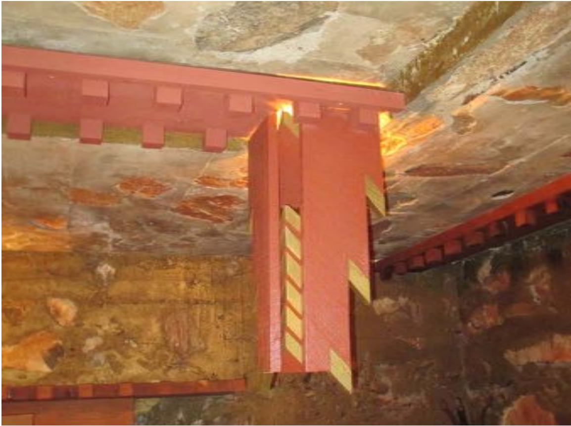
Figure 10-53 - Wood pendant light fixture in Kiva, 2014 (Harboe Architects).
