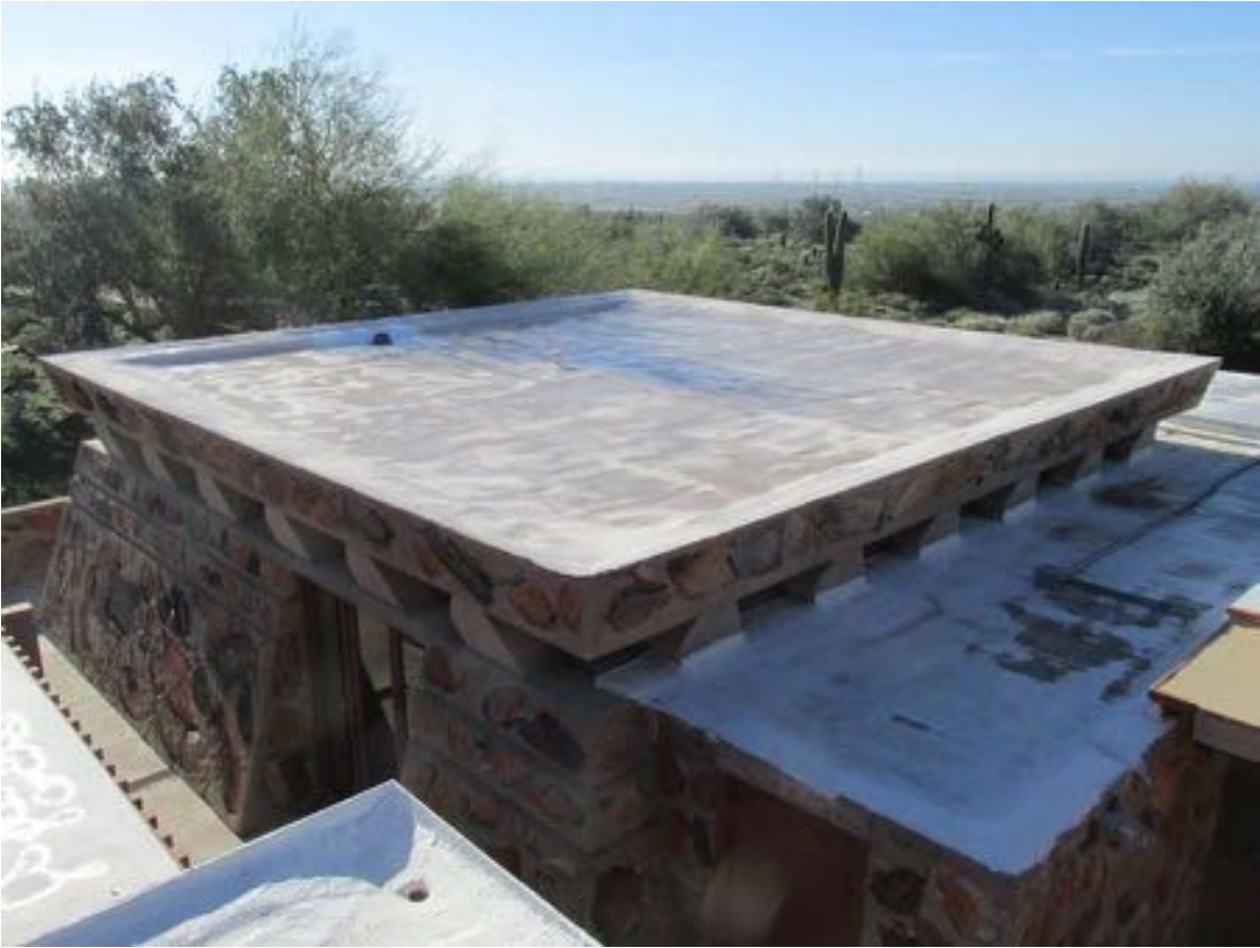
Figure 11-217 - Roof of Clinic Office, 2015 (Harboe Architects).
