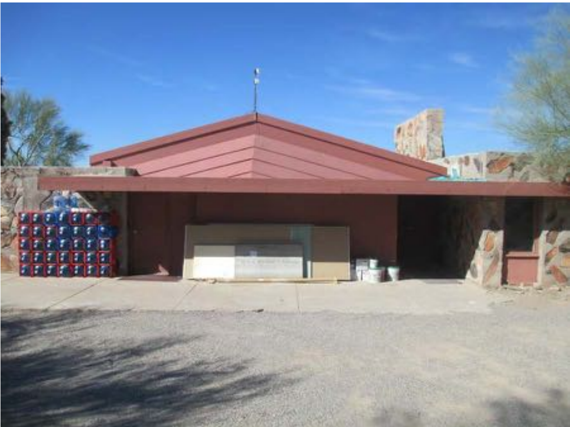
Figure 10-179 - East side of the Pavilion, 2014 (Harboe Architects).
