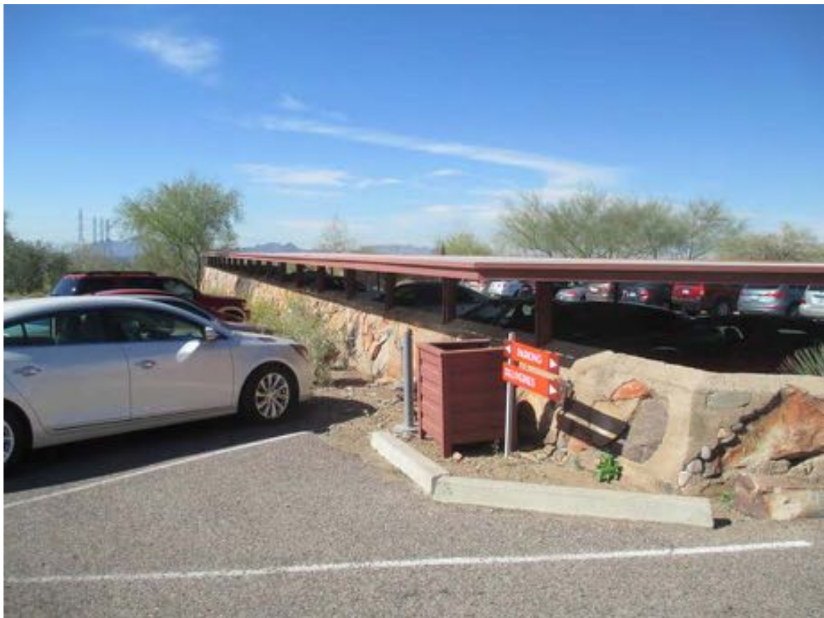
Figure 11-239 - Looking west at parking canopy, 2014 (Harboe Architects).
