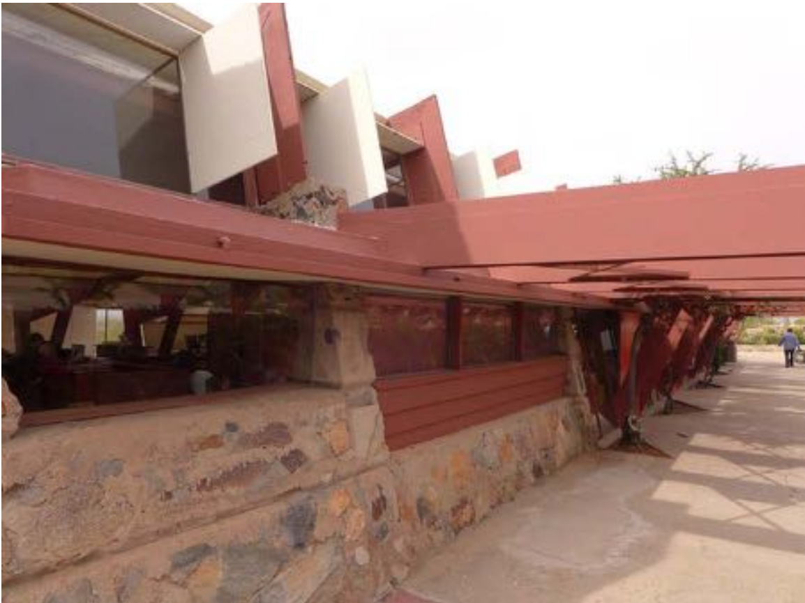
Figure 11-23 - Northwest side of Drafting Studio, 2014 (Harboe Architects).
