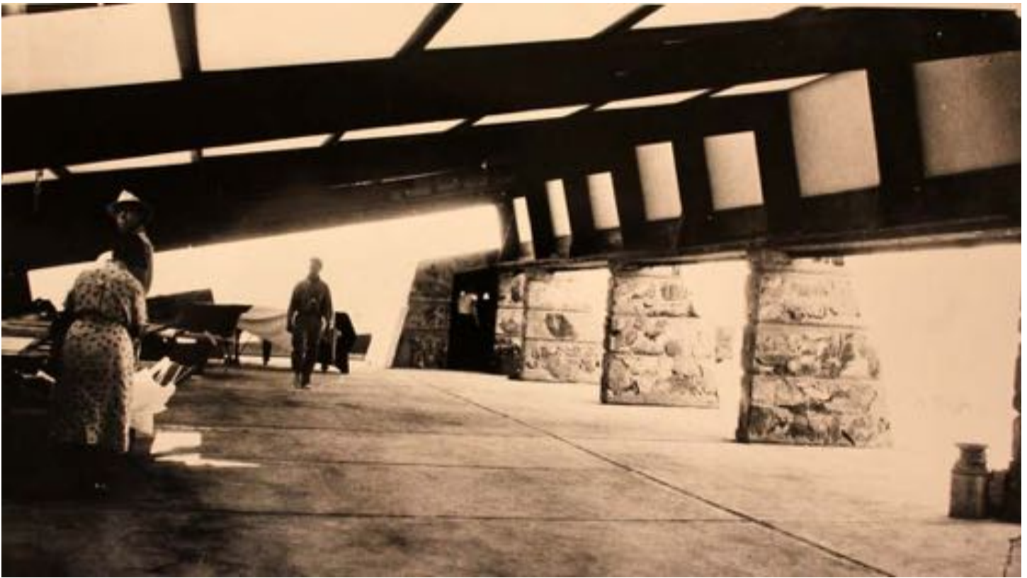
Figure 8-2 - Interior of the Drafting Studio looking west, ca. 1939 (The Frank Lloyd Wright Foundation Archives, The Museum of Modern Art | Avery Architectural & Fine Arts Library, Columbia University, New York).
