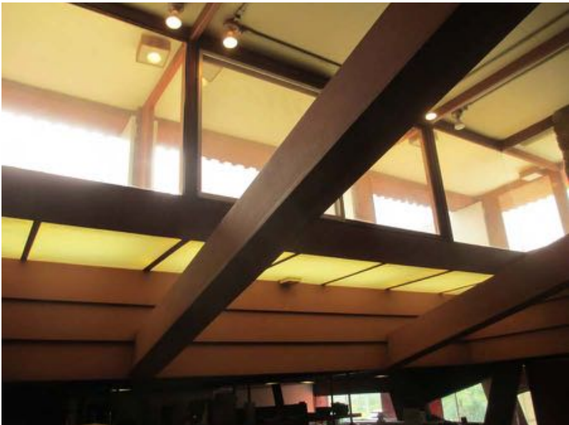
Figure 10-30 - Interior of Kitchen looking up at clerestory windows, 2014 (Harboe Architects).
