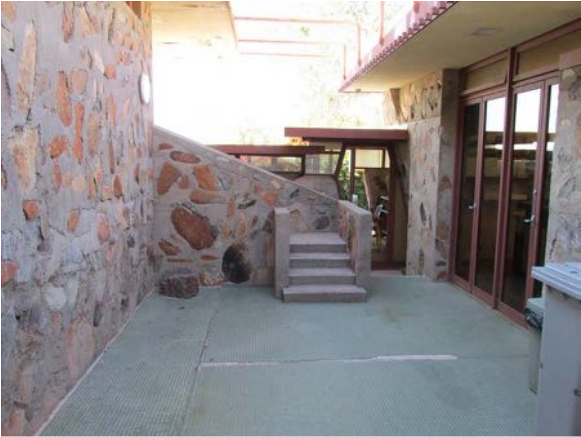
Figure 10-231 - Courtyard outside the Finance Office, 2015 (Harboe Architects).
