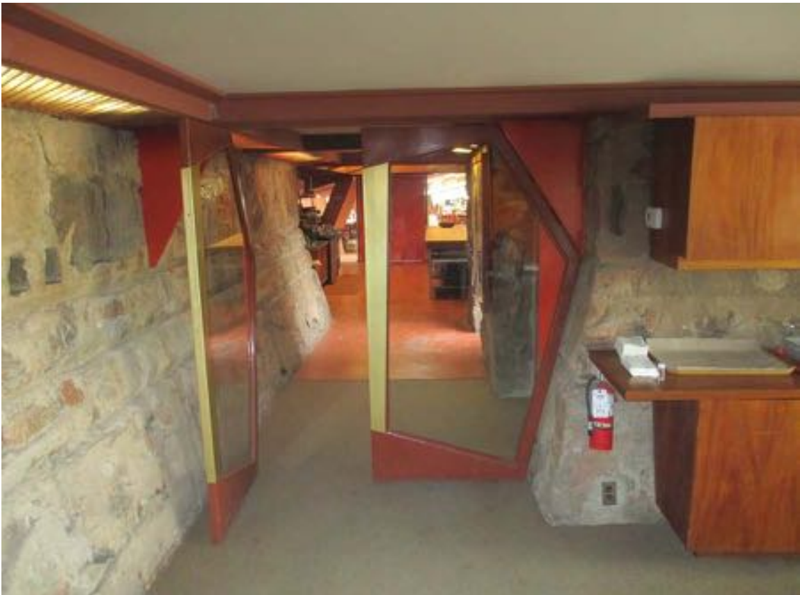
Figure 11-112 - Interior of Dining Room looking northwest at doors to kitchen, 2014 (Harboe Architects).
