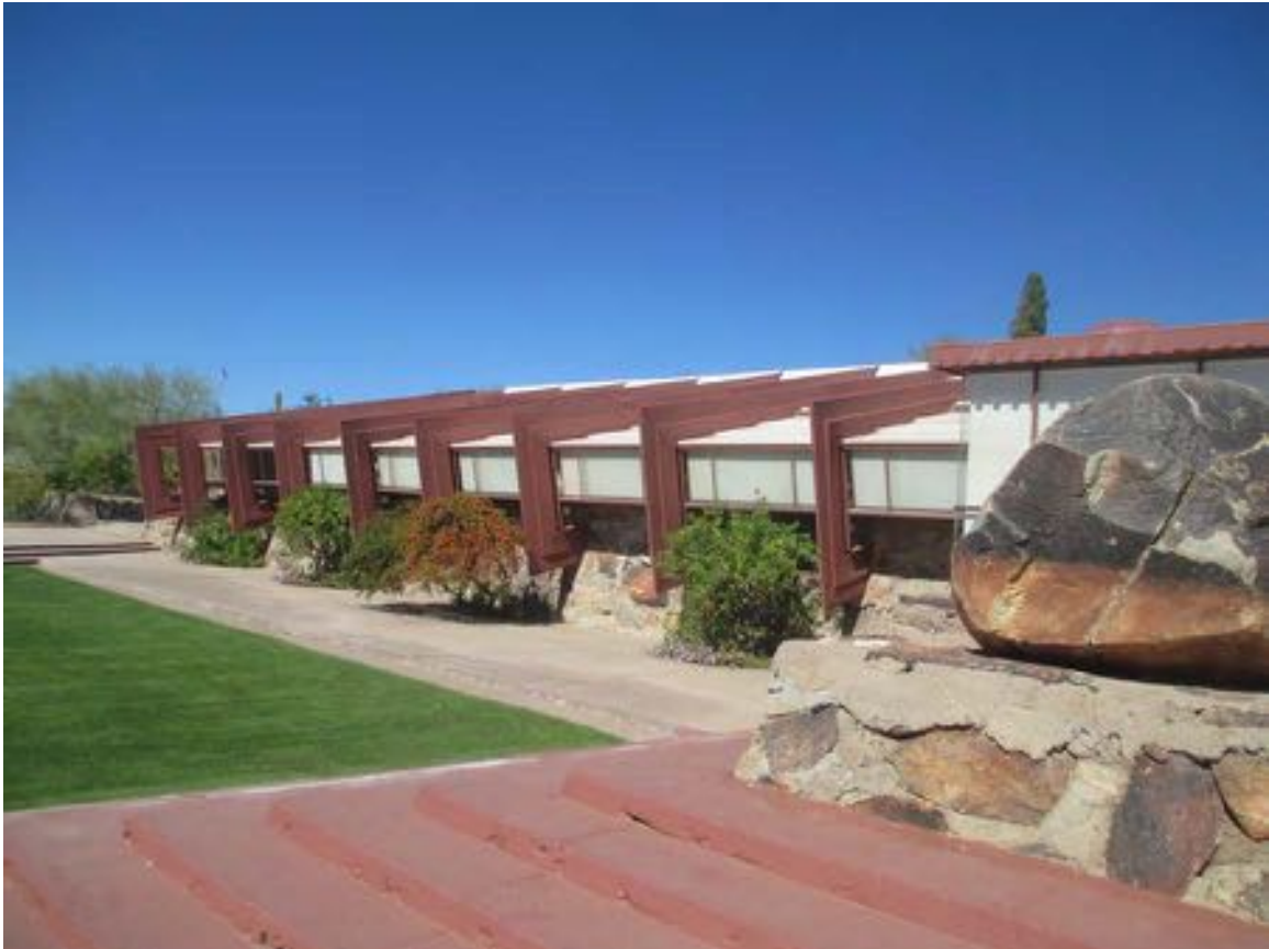
Figure 10-13 - Southeast side of Drafting Studio, 2014 (Harboe Architects).
