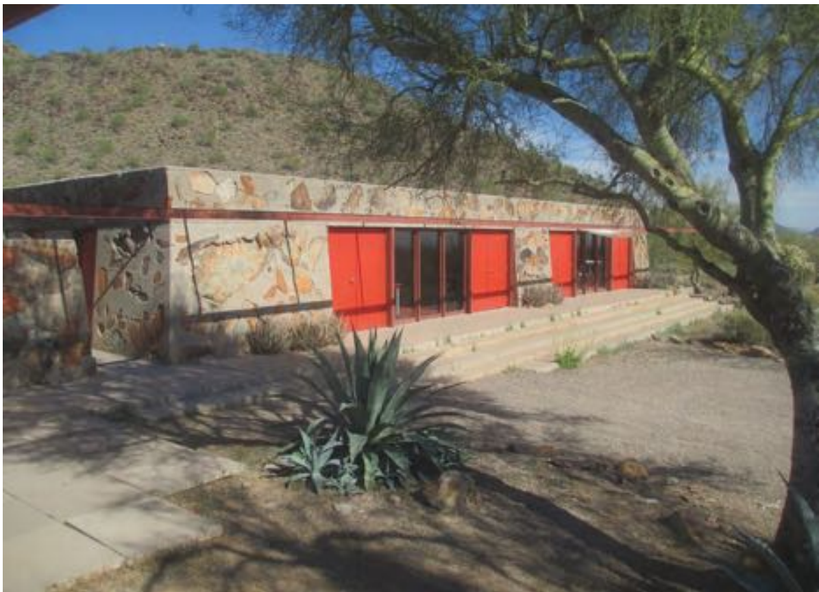
Figure 10-222 - Looking east at the East Wing, 2014 (Harboe Architects).
