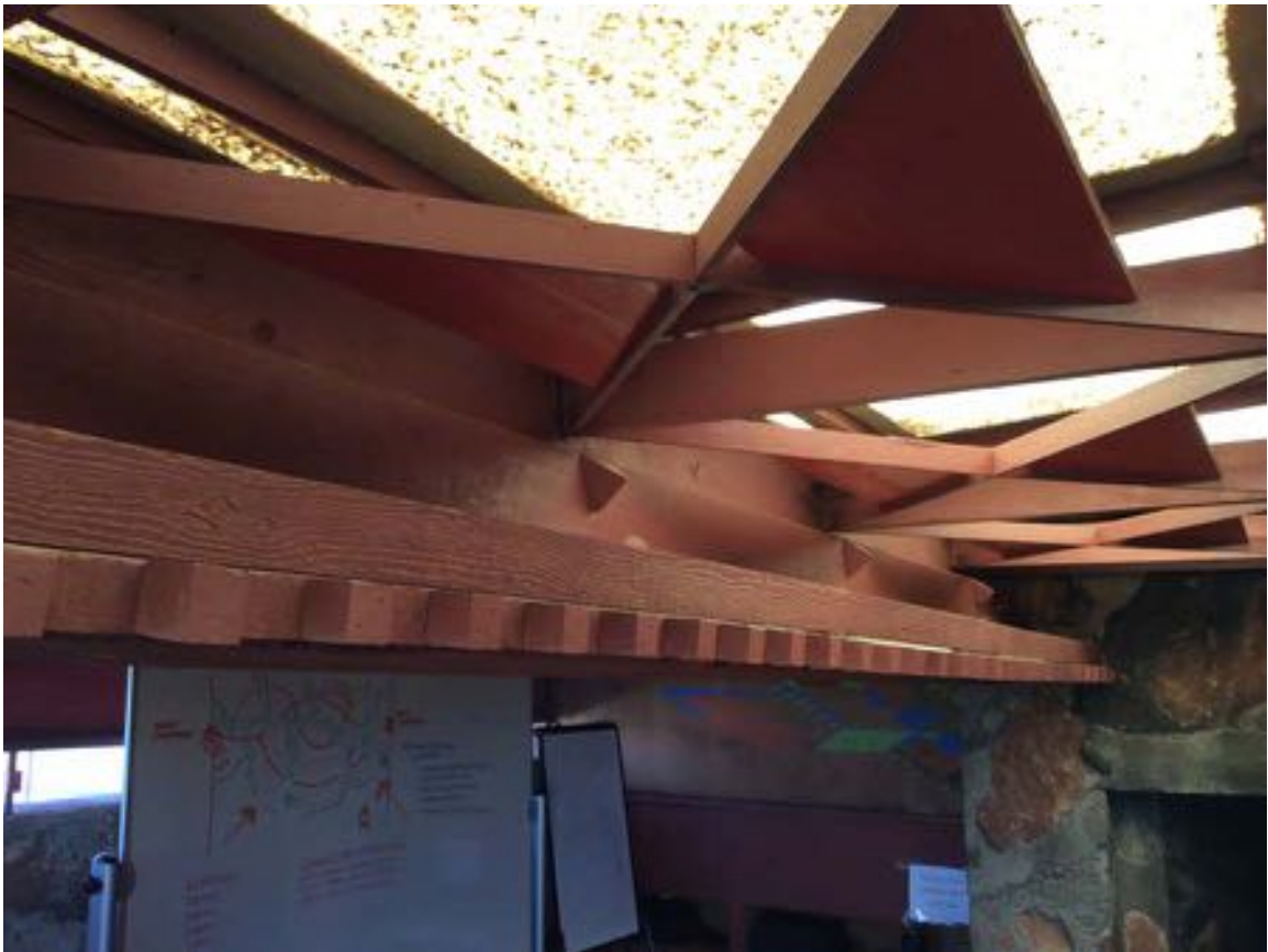
Figure 10-45 - Wood trellis work under the skylight, 2014 (Harboe Architects).
