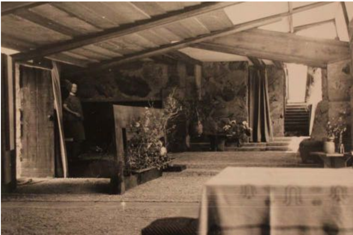
Figure 6-21 - Interior of Garden Room, ca. 1940 (The Frank Lloyd Wright Foundation Archives, The Museum of Modern Art | Avery Architectural & Fine Arts Library, Columbia University, New York).
