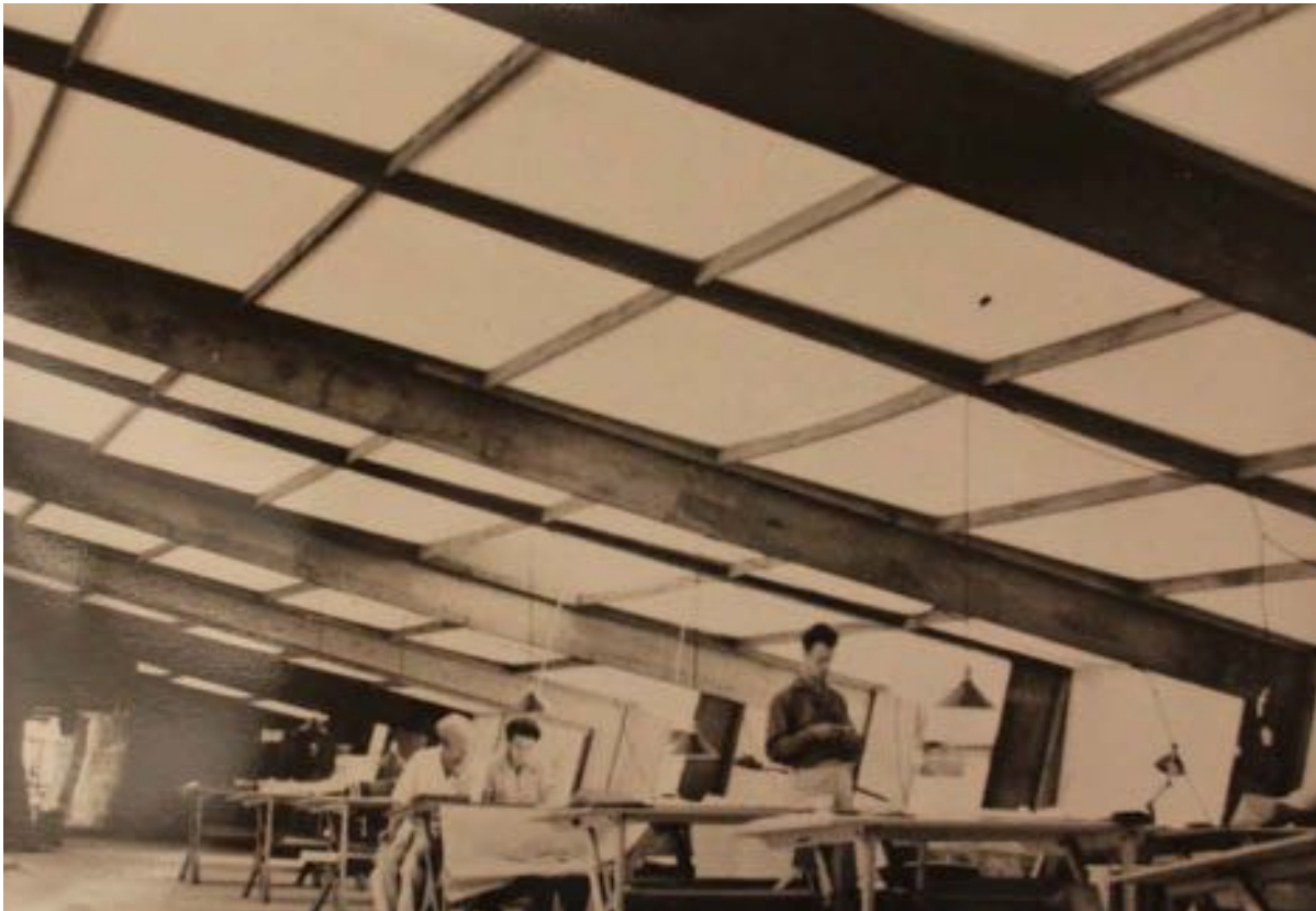
Figure 6-14 - Canvas roof overhead in Drafting Studio, ca. 1939 Drafting Studio (The Frank Lloyd Wright Foundation Archives, The Museum of Modern Art | Avery Architectural & Fine Arts Library, Columbia University, New York).
