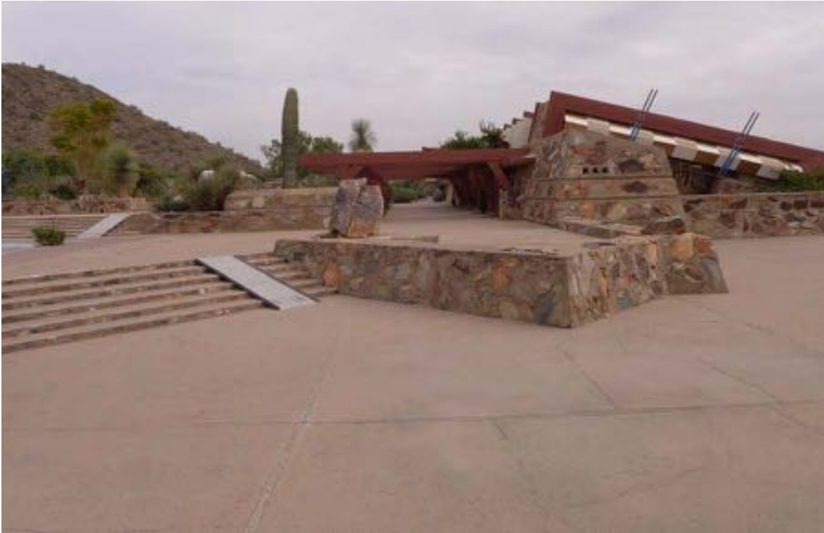
Figure 11-249 - Paved area between the office and Drafting Studio, 2014 (Harboe Architects).
