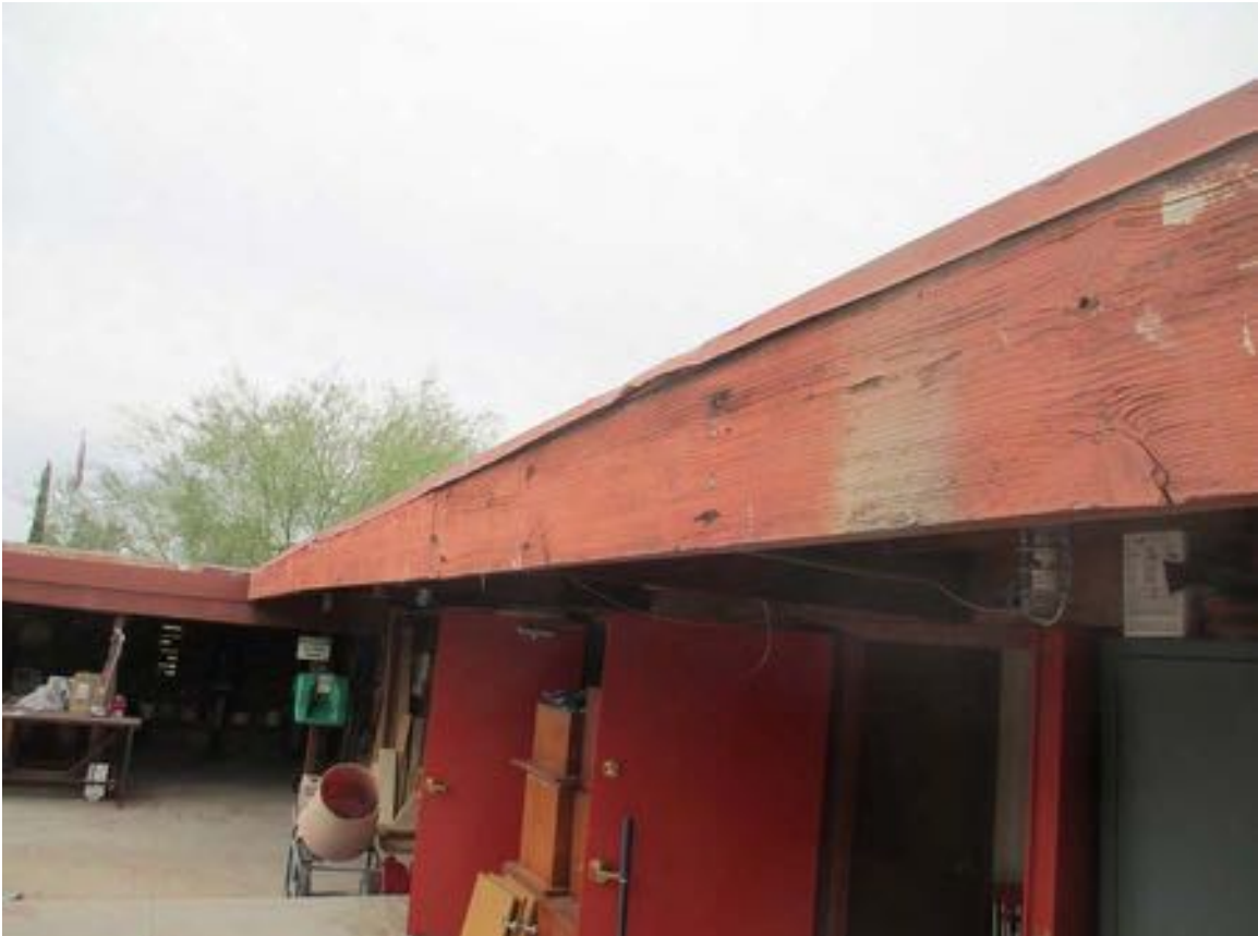
Figure 11-135 - View of Shops showing wood fascia at eaves, 2014 (Harboe Architects).
