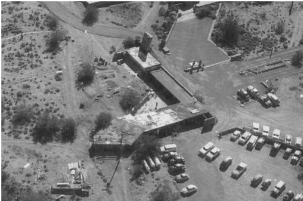
Figure 11-130 - Aerial view of the Shops, ca 1959 (The Frank Lloyd Wright Foundation Archives, The Museum of Modern Art | Avery Architectural & Fine Arts Library, Columbia University, New York).
