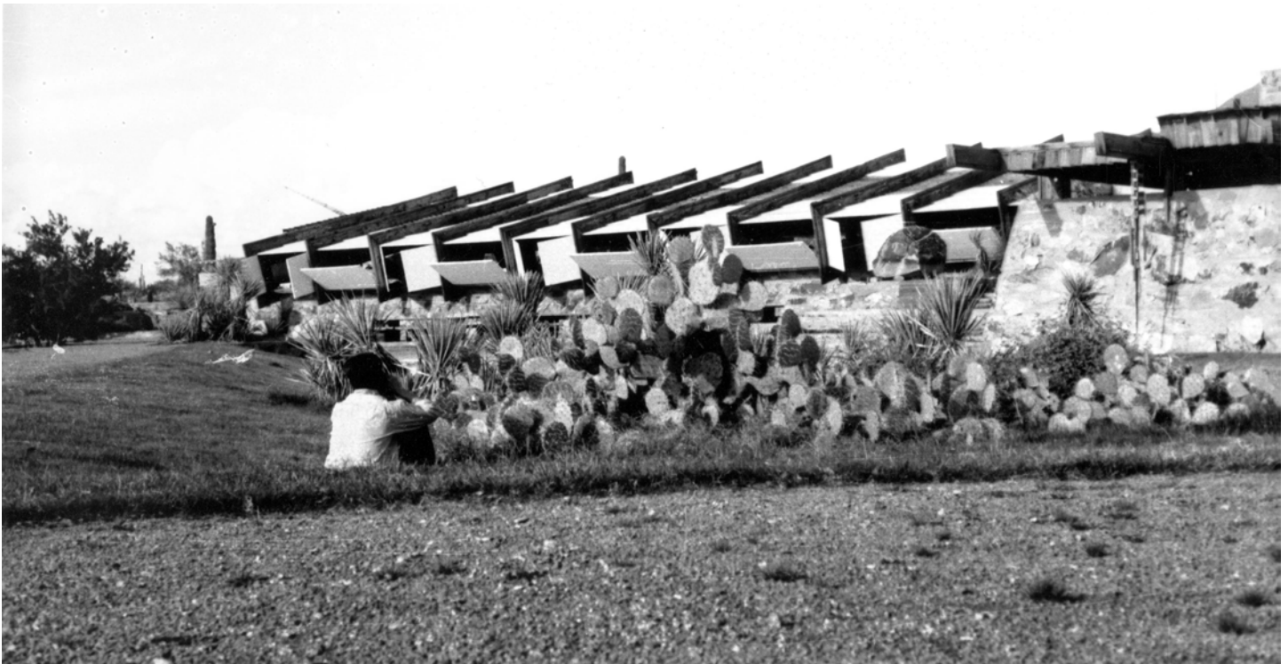
Figure 7-101 - Desert plantings on prow in front of Drafting Studio, ca. 1941 (The Frank Lloyd Wright Foundation Archives, The Museum of Modern Art | Avery Architectural & Fine Arts Library, Columbia University, New York).
