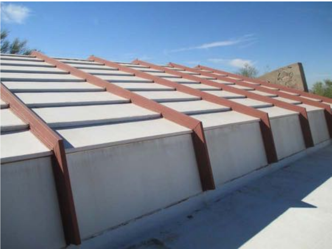
Figure 10-177 - Pavilion roof, 2014 (Harboe Architects).
