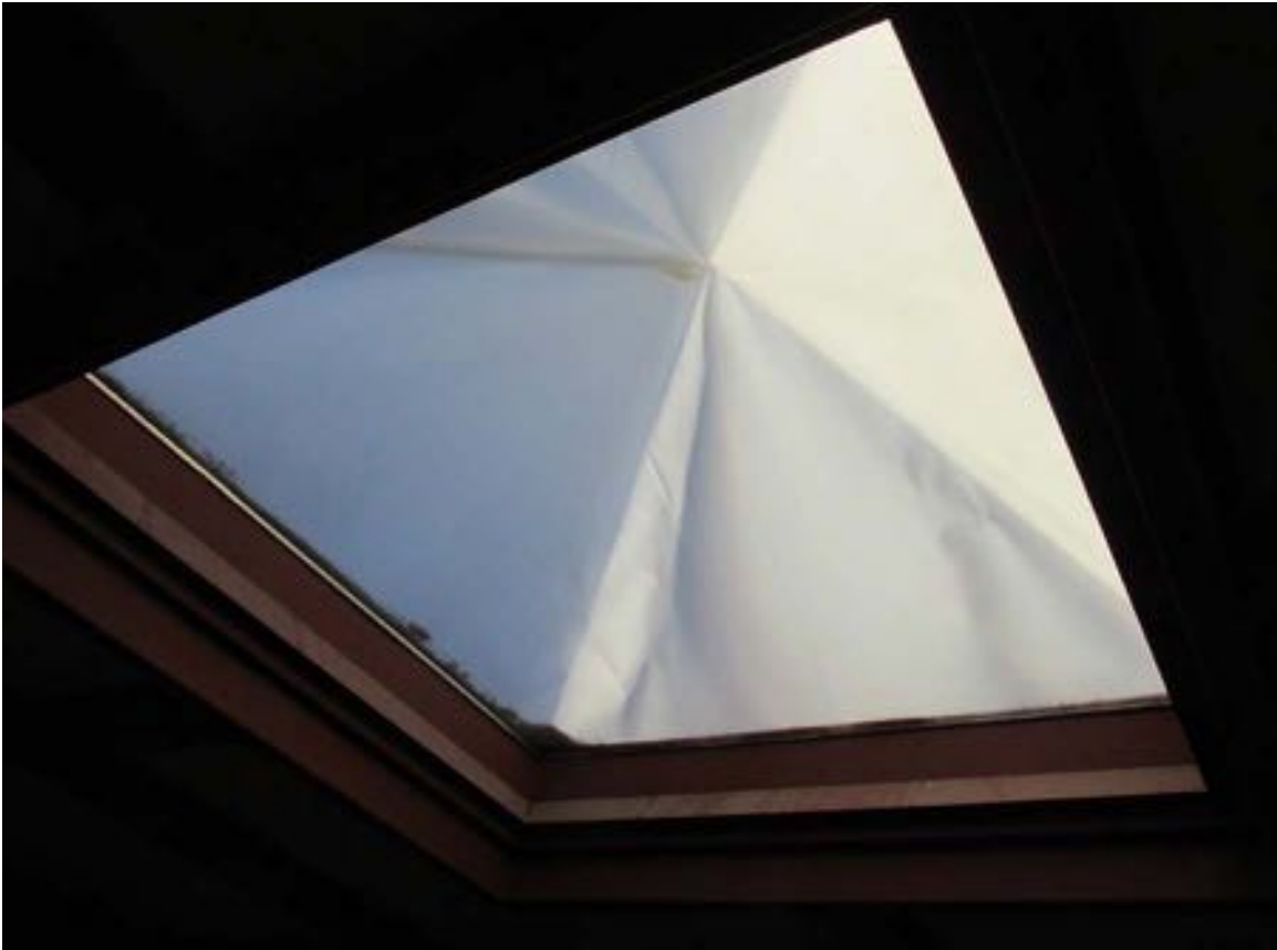
Figure 10-212 - Atrium skylight, 2014 (Harboe Architects).
