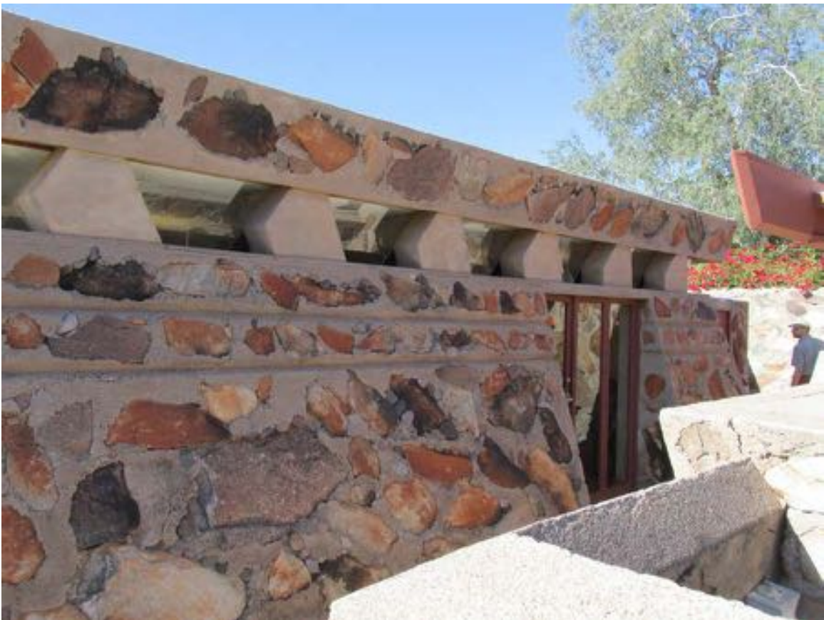
Figure 10-268 - North facade of Clinic Office, 2015 (Harboe Architects).
