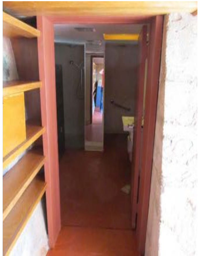
Figure 10-249 - Looking into bathroom, 2015 (Harboe Architects).
