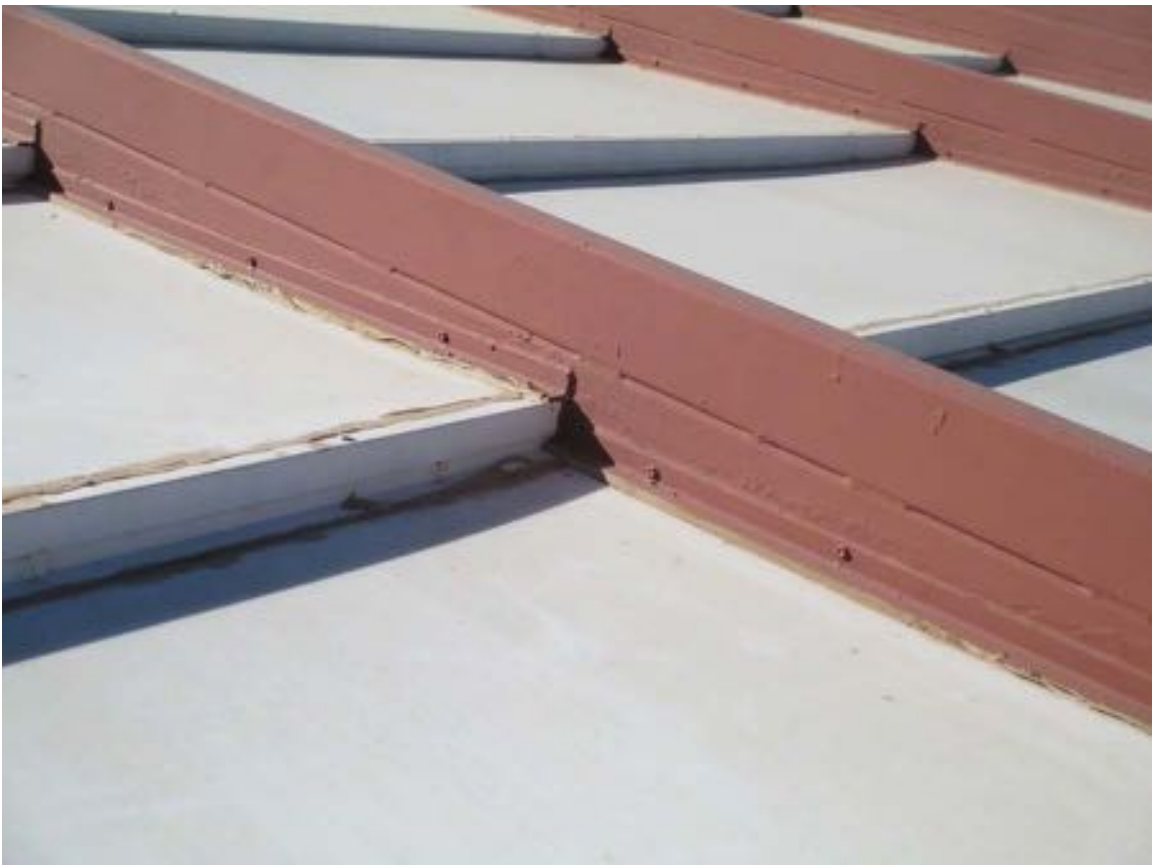
Figure 11-161 - Detail of Pavilion roof, 2014 (Harboe Architects).
