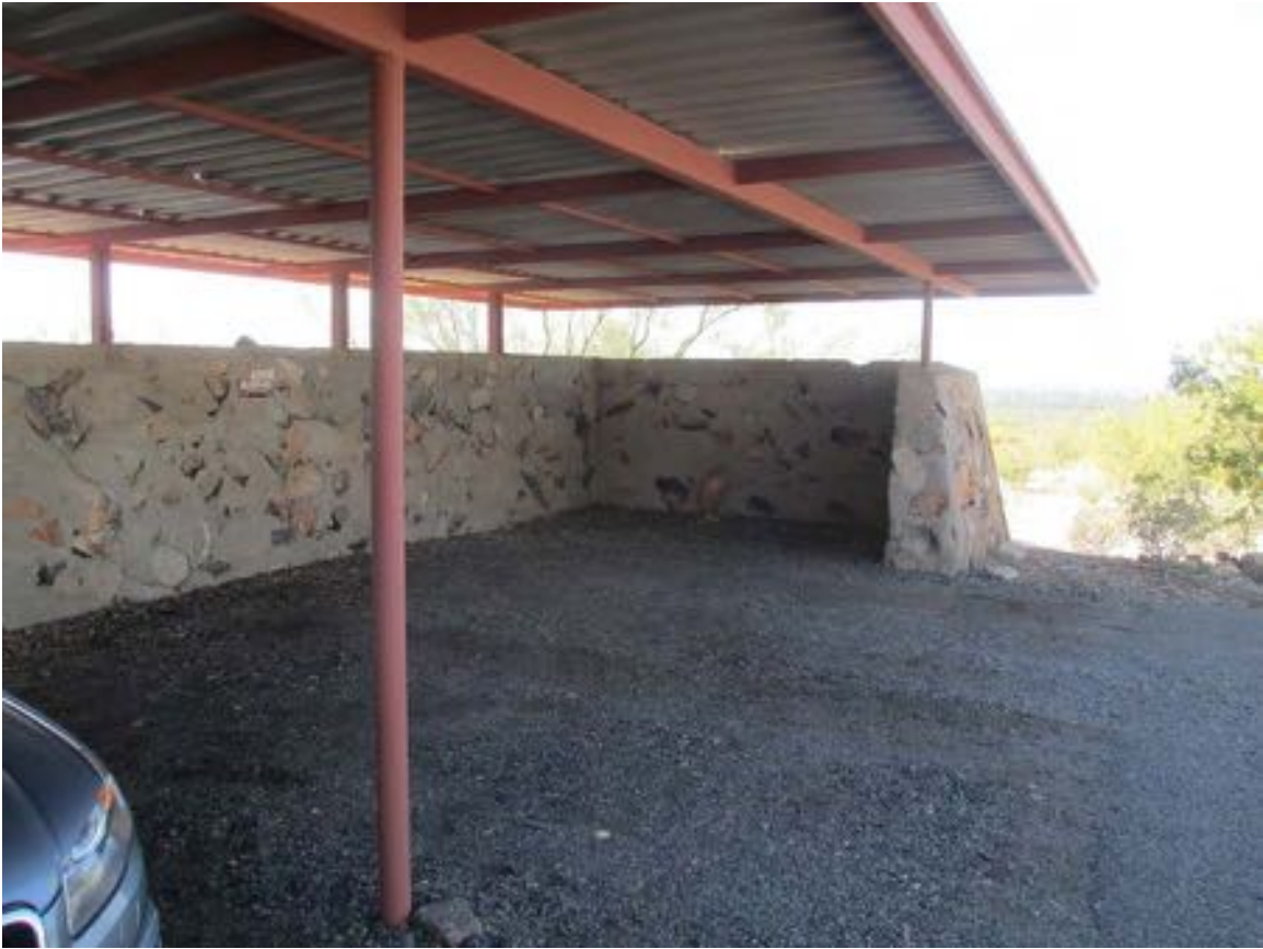
Figure 11-240 - Parking canopy and wall, 2014 (Harboe Architects).
