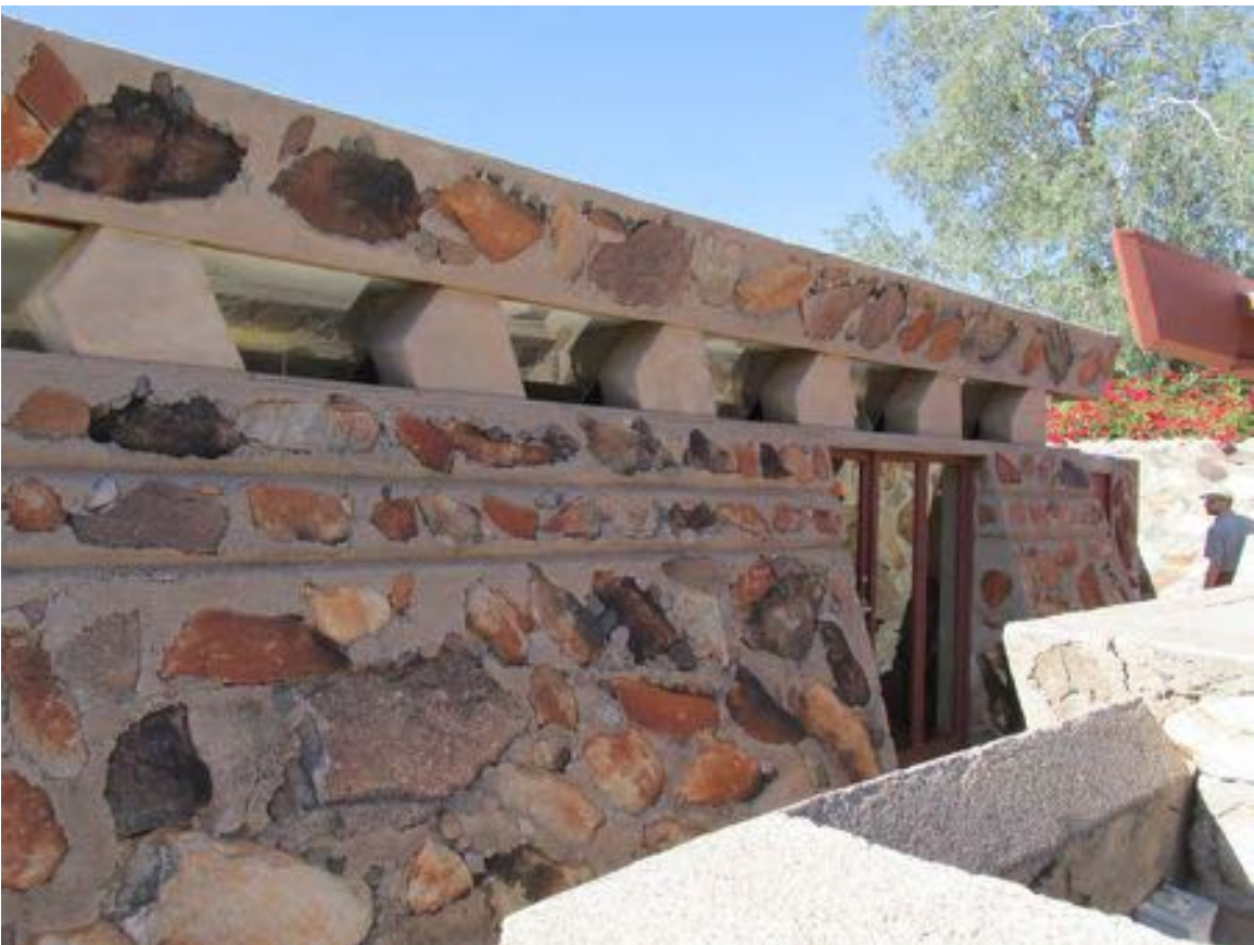
Figure 11-218 - North facade of Clinic Office, 2015 (Harboe Architects).
