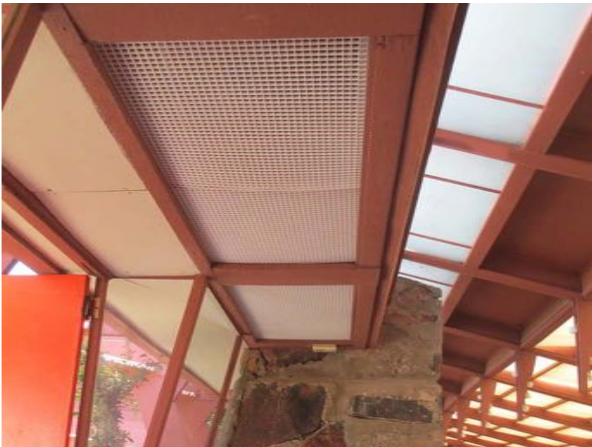
Figure 10-26 - Soffit under north clerestory, 2014 (Harboe Architects).
