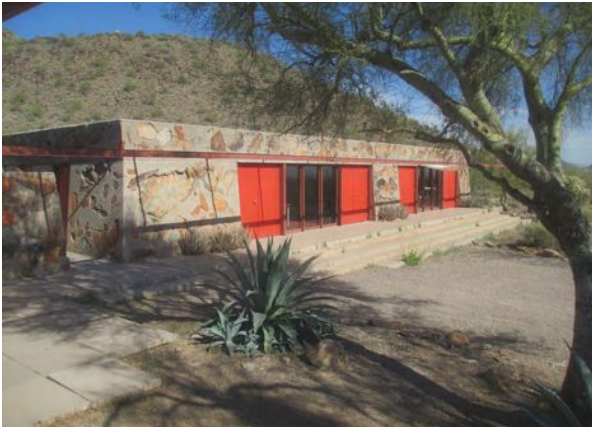
Figure 11-185 - Looking east at the East Wing, 2014 (Harboe Architects).
