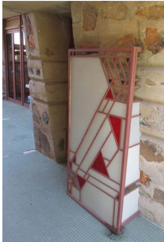
Figure 11-194 - Metal and glass gate at opening to courtyard outside of Finance Office, 2015 (Harboe Architects).
