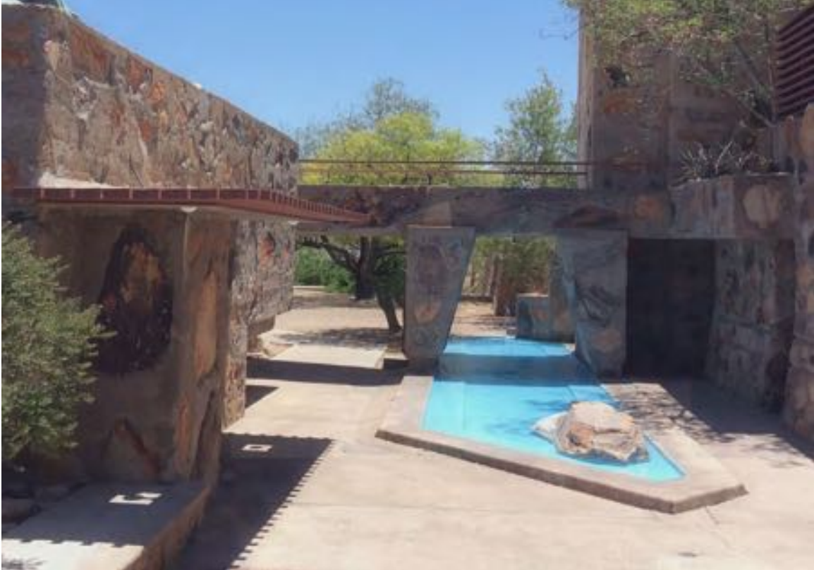
Figure 11-263 - Small pool under Kiva Bridge, 2014 (Harboe Architects).
